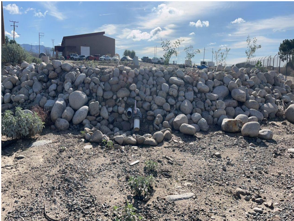
Figure 6. General View of Granite Boulders, Foothill Pump Station Building and a Plastic Pipe Feature, View SE
