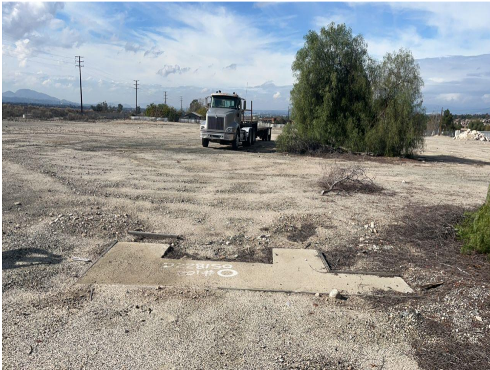
Figure 7. General View of F-Shape Poured Cement Foundation, View SW
