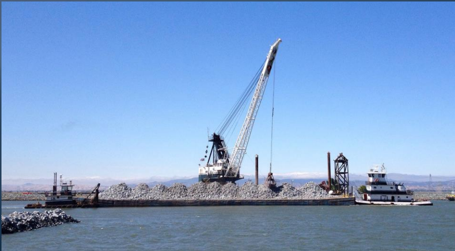
Emergency Drought Barrier Installation in 2015
