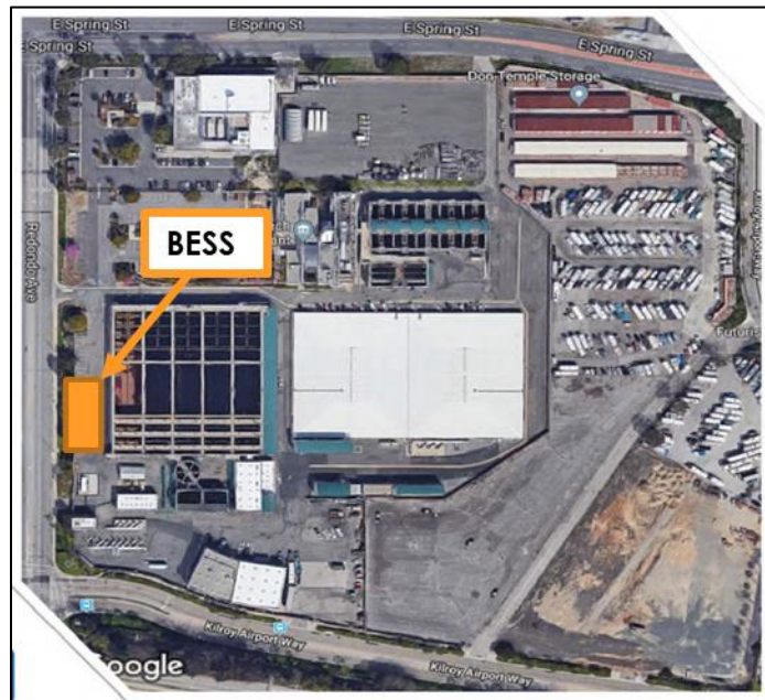
Figure A-1. Aerial view of the LBWD's BESS.
