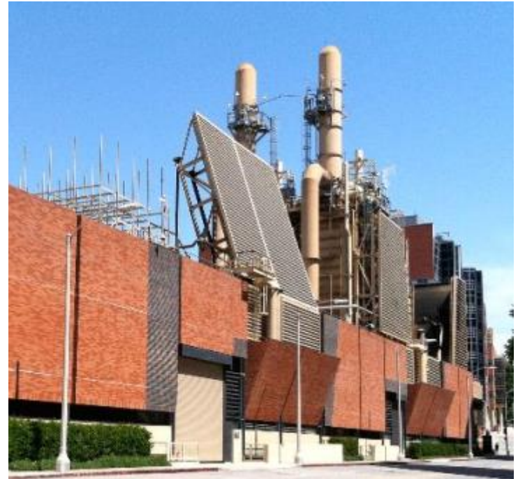
UCLA Cogeneration Plant
