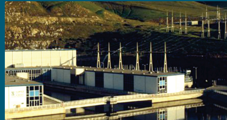
Edmonston Pumping Plant "Big Lift"
