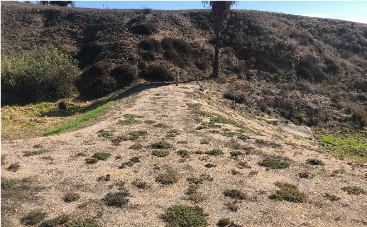
Photograph 5. Berm above culvert separating Basin 1 from Basin 2, facing southeast.
