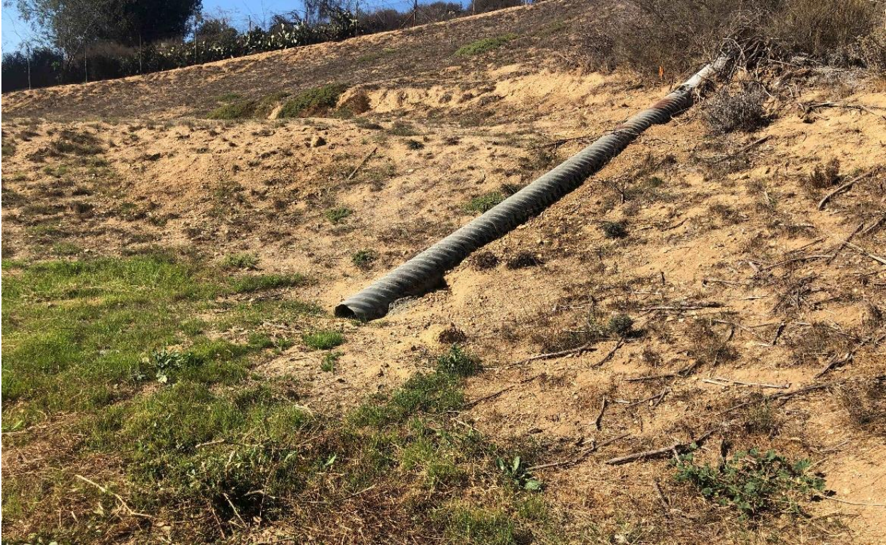
Photograph 3. Corrugated pipe conveying runoff into Basin 1, facing west.
