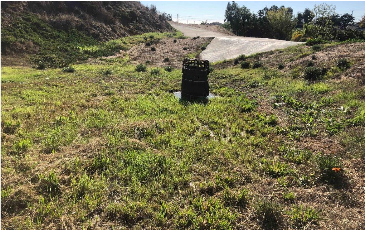
Photograph 8. Inlet drain receiving flow from Basin 2, facing east-southeast.
