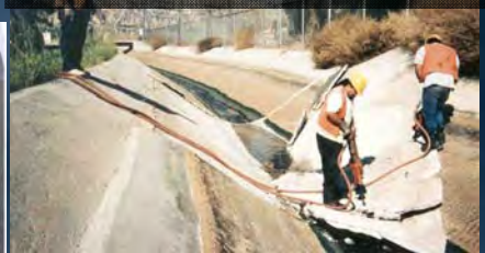
Channel dike failure, internal erosion (delayed), 1994 Northridge Earthquake
