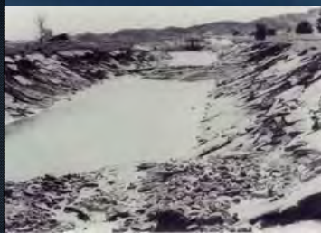
Channel failure, differential ground movement & erosion, 1971 San Fernando Earthquake
