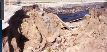
Channel dike failure, internal erosion (delayed), 1994 Northridge Earthquake
