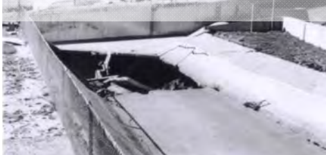
Channel failure, differential ground movement & erosion, 1971 San Fernando Earthquake
