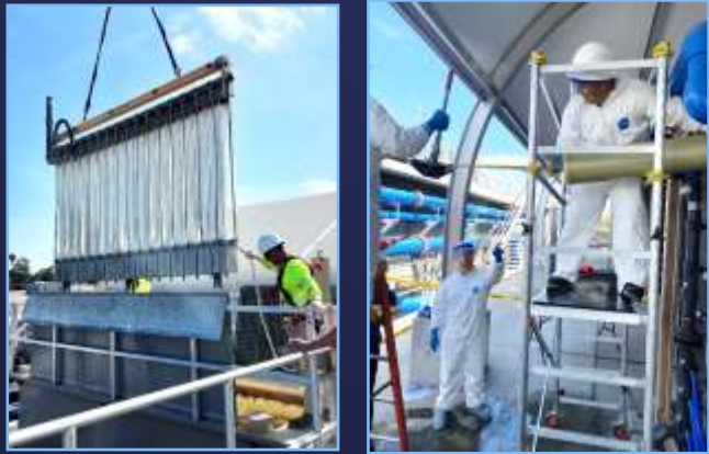
Replacement of membranes
