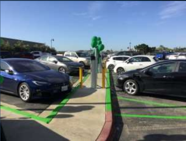
EV Charging Stations
