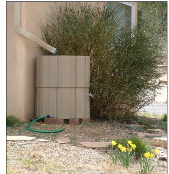
Smaller cisterns or rain barrels can be used to capture and reuse residential rooftop runoff for irrigation and other non-potable uses.
