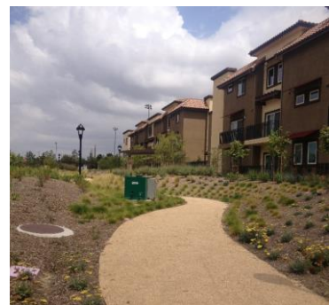
Underground Cistern Taylor Yard
