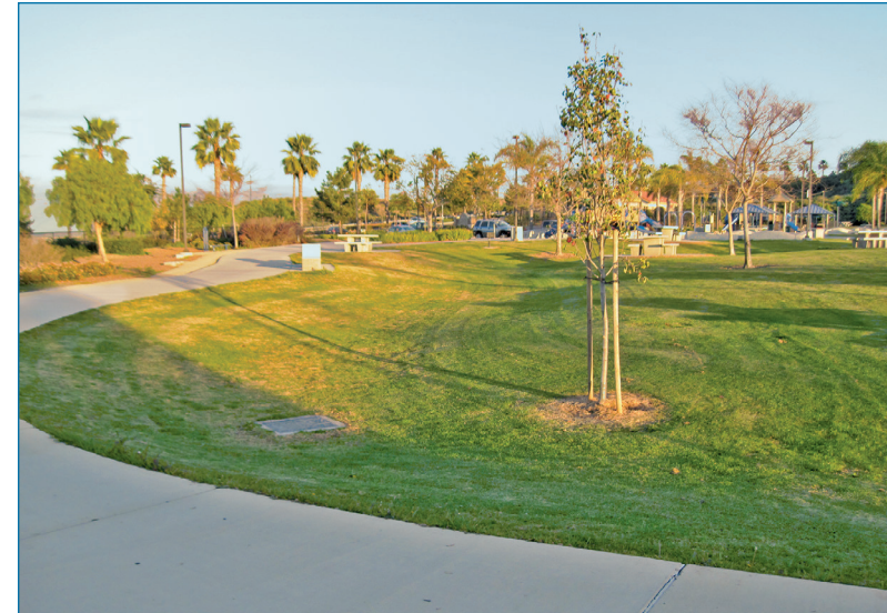
A vegetated swale conveys and treats runoff from a public park. Proper design, maintenance of dense vegetation, and accurate fine grading ensure optimum treatment and minimize the risks of erosion or standing water.
