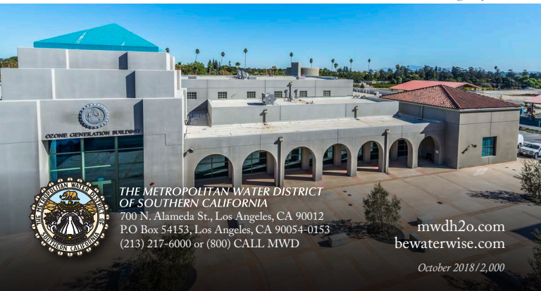
Ozone Generation Building, Weymouth
