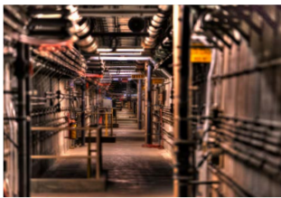
Diemer Water Treatment Plant
