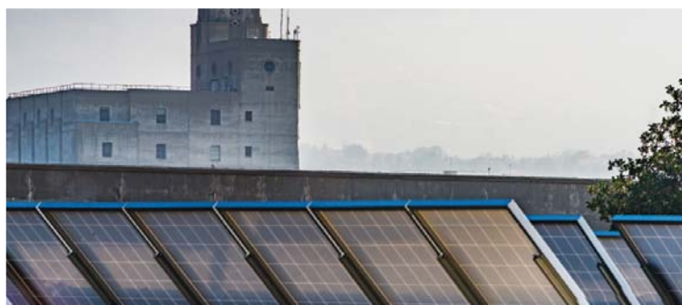
WEYMOUTH WATER TREATMENT PLANT IN LA VERNE
