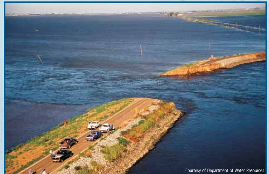
California was reminded of the fragility of the Bay-Delta system with this 2004 levee break at Jones Tract.
