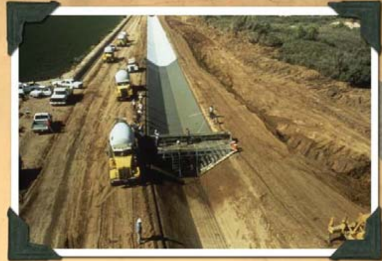
LINING CANALS TO SAVE WATER
