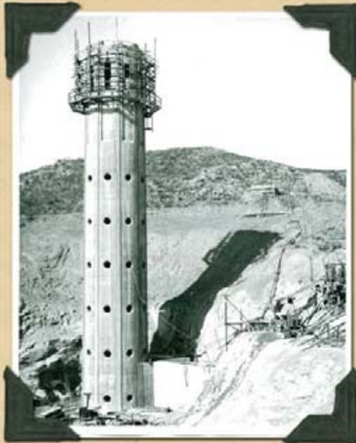
ORIGINAL LAKE MATHEWS OUTLET TOWER
