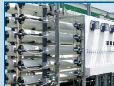
City of Long Beach Water Department developed a two-stage nanofiltration process to remove salt from seawater while using about one-third less energy than traditional desalination.
