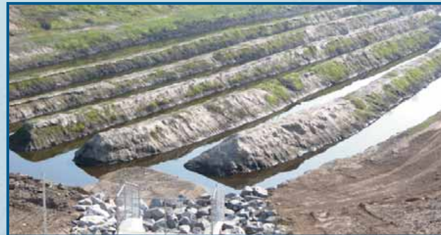
This Chino Basin recharge field naturally treats water so it can be used beneficially.
