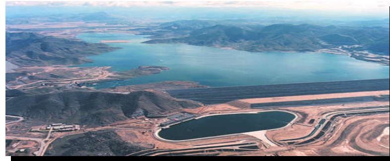
West Dam View of Diamond Valley Lake (DVL), the Southland’s newest and largest reservoir. When completely filled, DVL will double the storage capacity for Southern California and provide six months of emergency supply.
