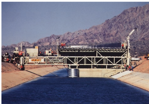
Lining the Coachella Canal with concrete.
