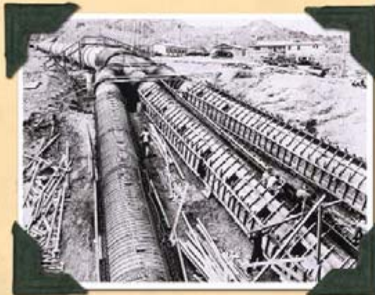
EARLY PIPELINE CONSTRUCTION
