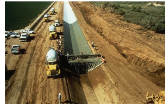
Canal lining in the Imperial Irrigation District.
