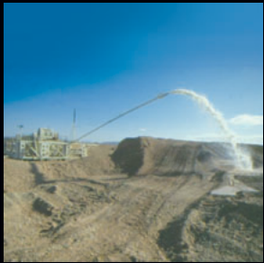
Coachella Canal Lining Project
