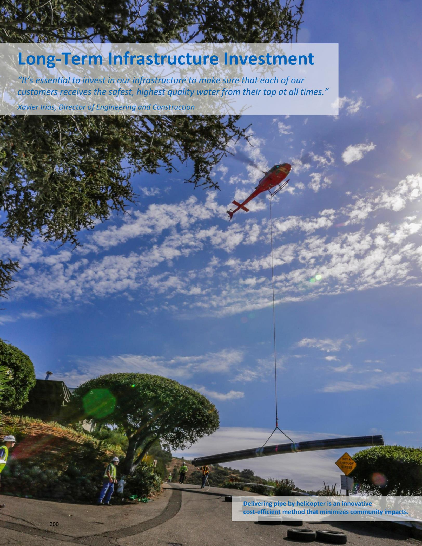
Delivering pipe by helicopter is an innovative cost-efficient method that minimizes community impacts.
