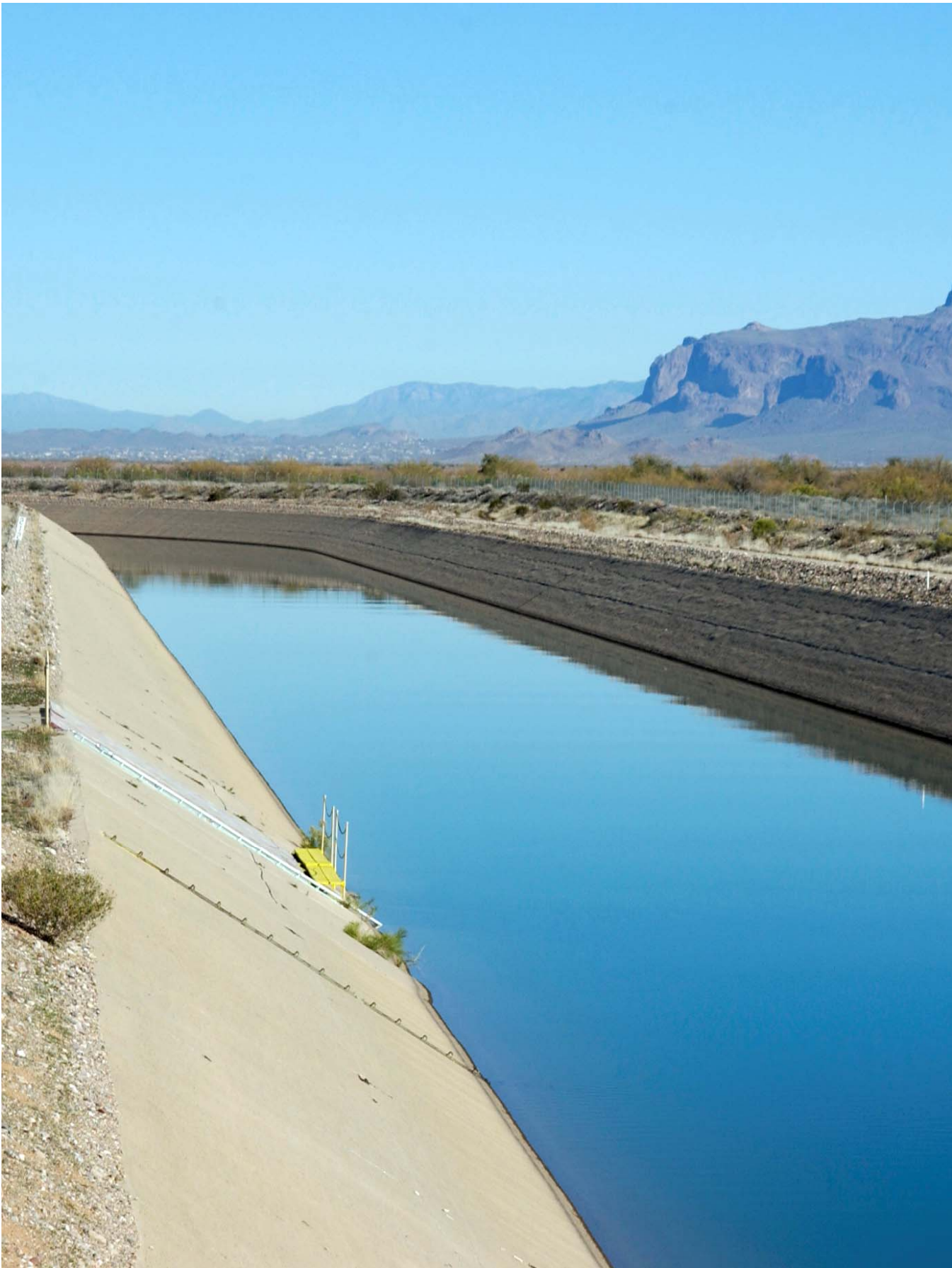
Aqueduct Maintenance South
