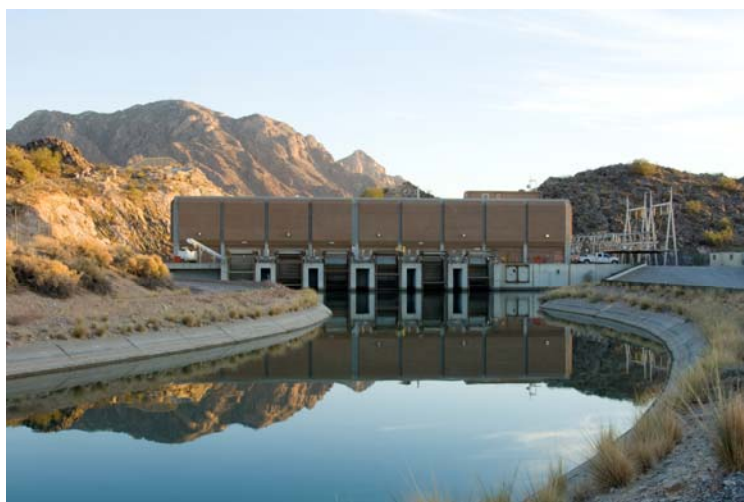
Picacho Pumping Plant
