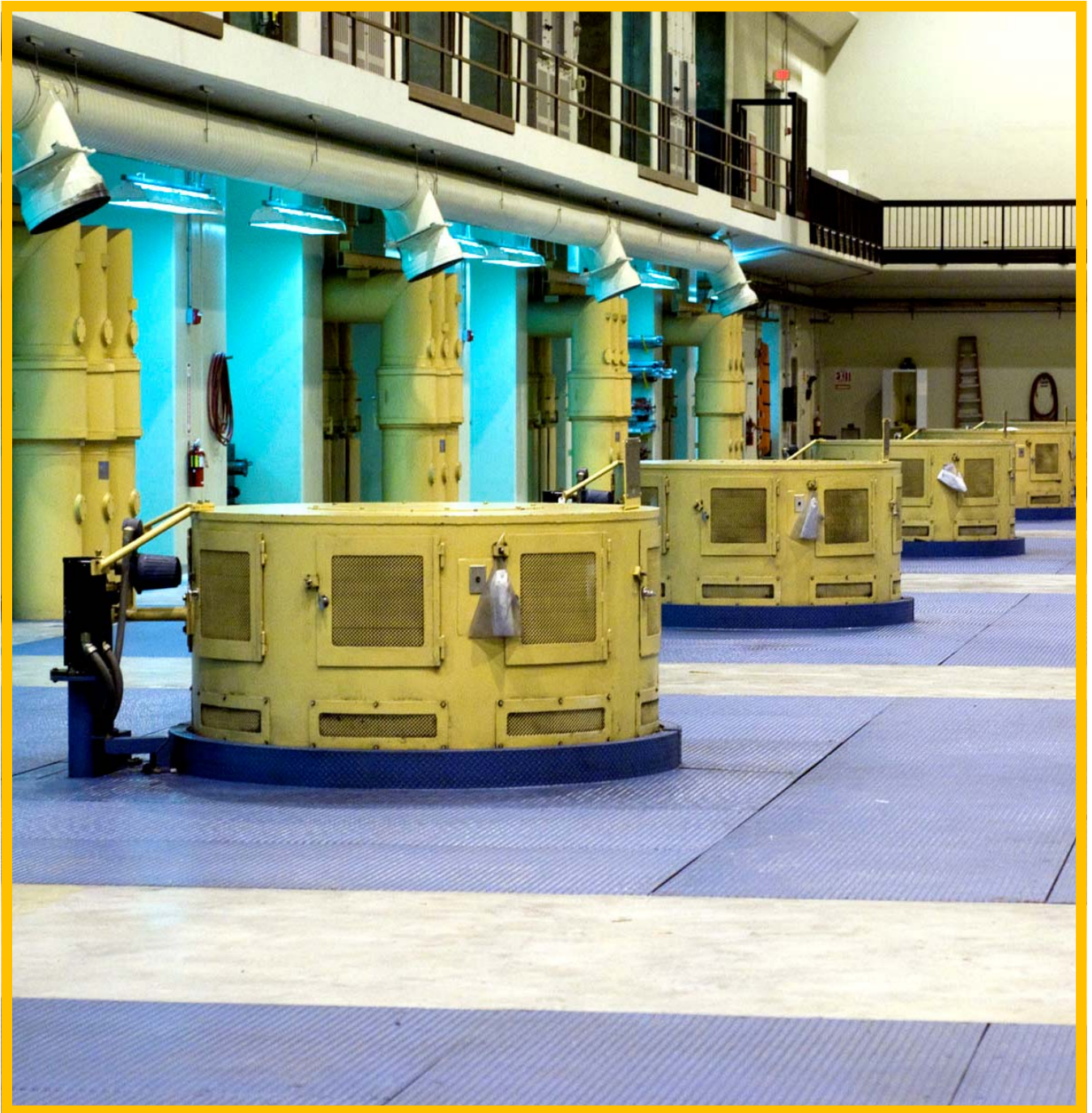
Inside Mark Wilmer Pumping Plant
