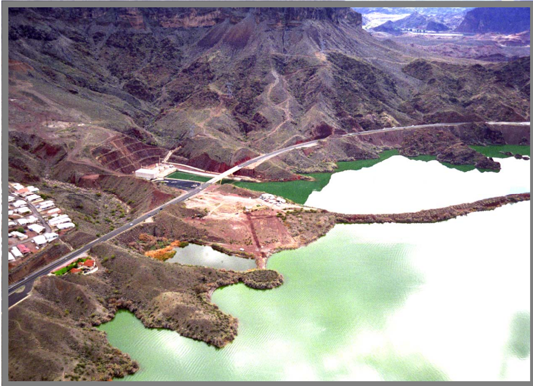
Mark Wilmer Pumping Plant Shoreline
