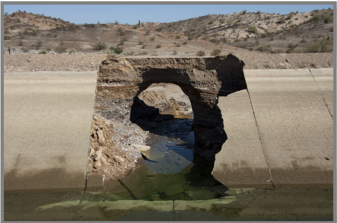
Canal Breach Mile Post 75
