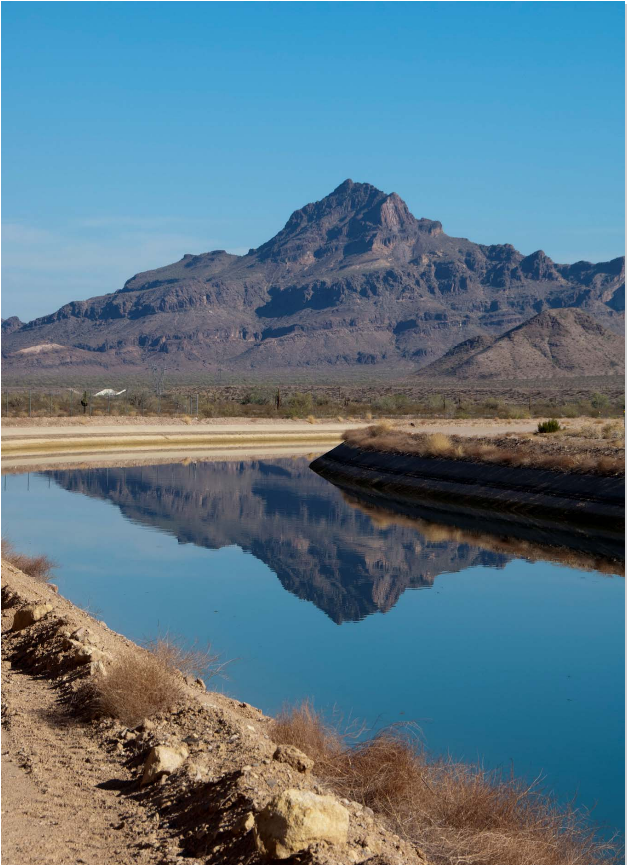
Burnt Mountain Conduit Install
