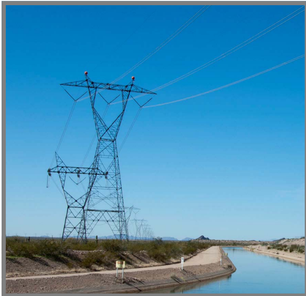
Power lines crossing canal
