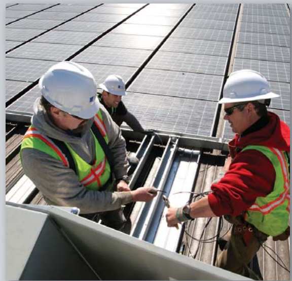
Solar panels installation at Pier 96
