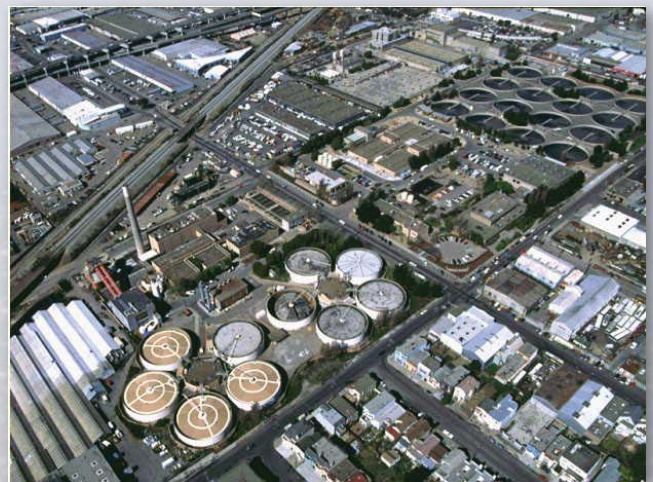
Southeast Wastewater Treatment Plant
