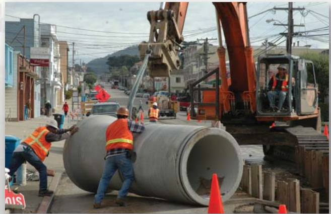
Vicente St. sewer construction project
