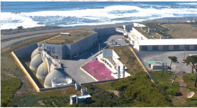
Oceanside Wastewater Treatment Plant
