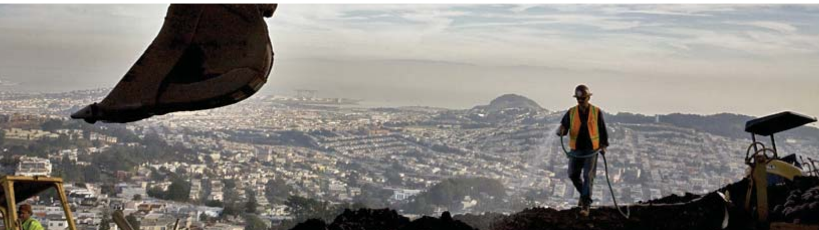
Worker at Mt. Davidson Tank
