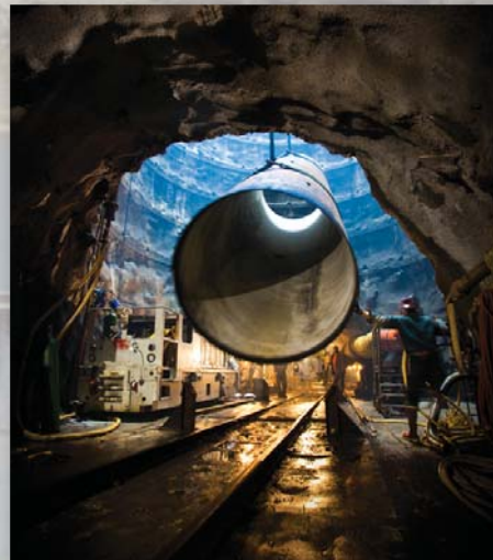
Construction on New Crystal Springs Bypass Tunnel
