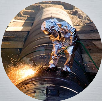
Construction on Bay Division Pipelines Nos. 3 & 4 Crossovers
