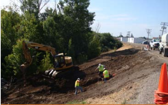
A District crew repairs a levee on the Guadalupe River.
