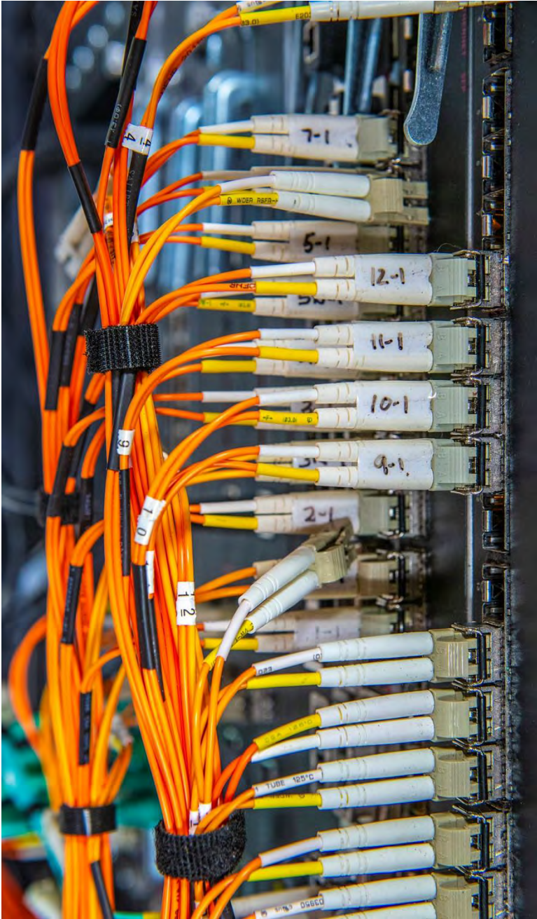
Fiber-optic cables connected to servers located inside the Data Center at Metropolitan's Headquarters.
