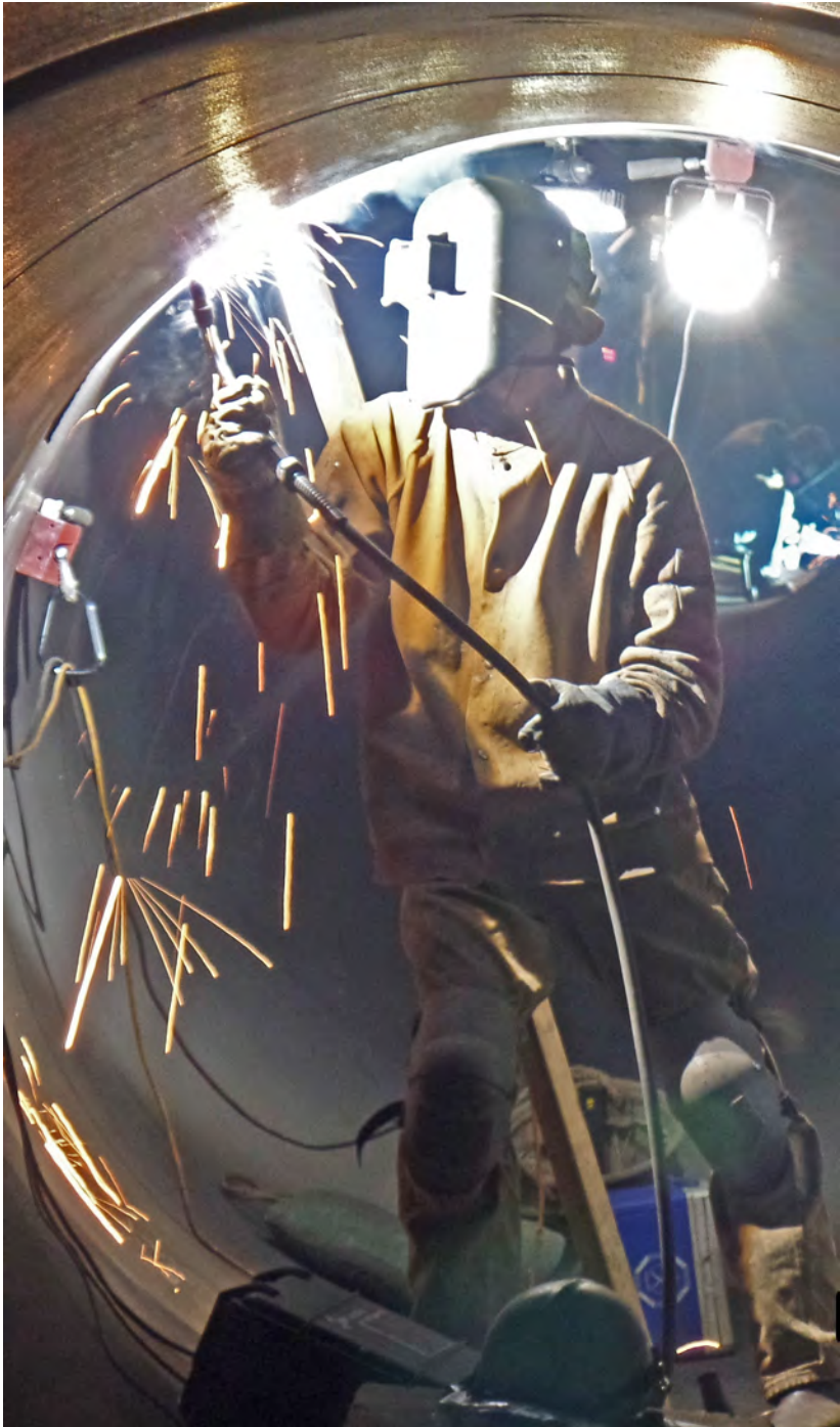
Welding joints on the steel liner of the Second Lower Feeder while rehabilitating prestressed concrete cylinder pipe.
