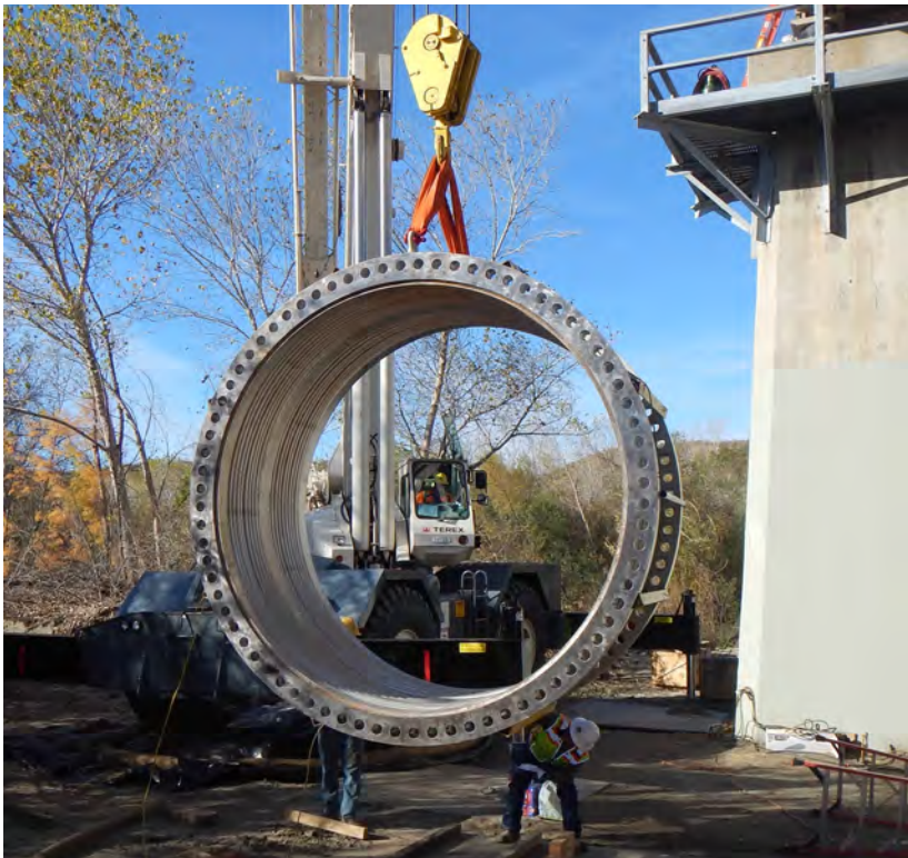
Installing an expansion joint on the Santa Ana River Bridge.
