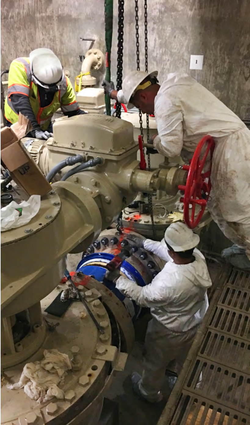
Staff reinstalling a pipe coupling at a pressure control structure on the Orange County Feeder.
