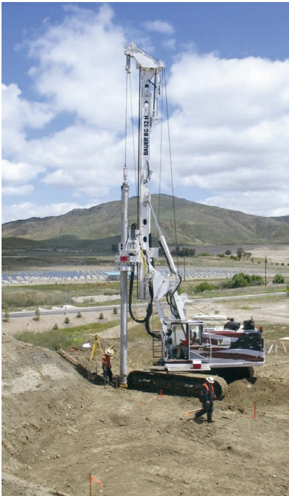
Drilling work to allow excavation of the Lake Skinner Outlet Conduit for repair work.
