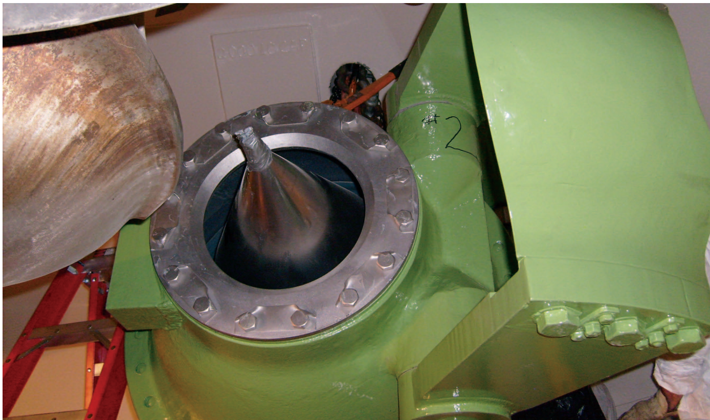
A refurbished turbine nozzle at the San Dimas Hydroelectric Plant.
