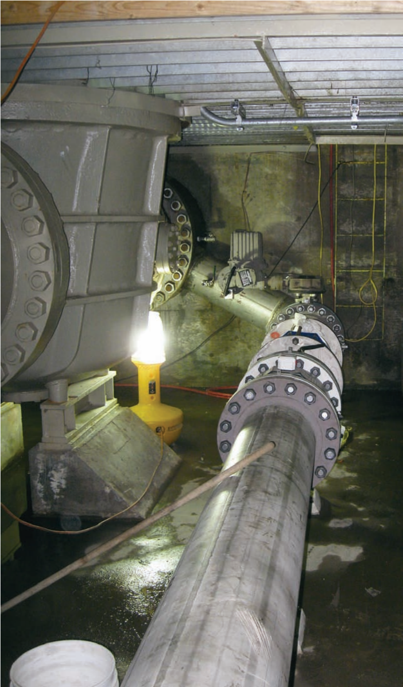
New piping and meter installation on Metropolitan's West Coast Feeder in the city of El Segundo.
