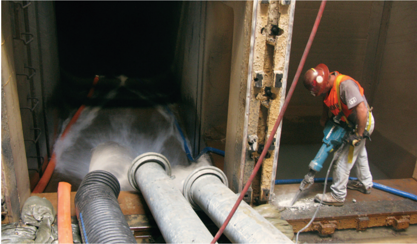
Pipes divert water from the West Portal of the San Jacinto Tunnel to accommodate rehabilitation work.
