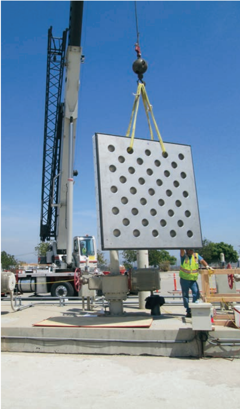
A crane hoists a multi-nozzle gate at the Jensen Water Treatment Plant effluent, May 2014.
