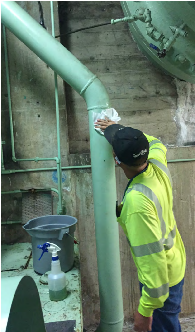
A student intern cleans an oil sump vent pipe at Gene Pumping Plant.
