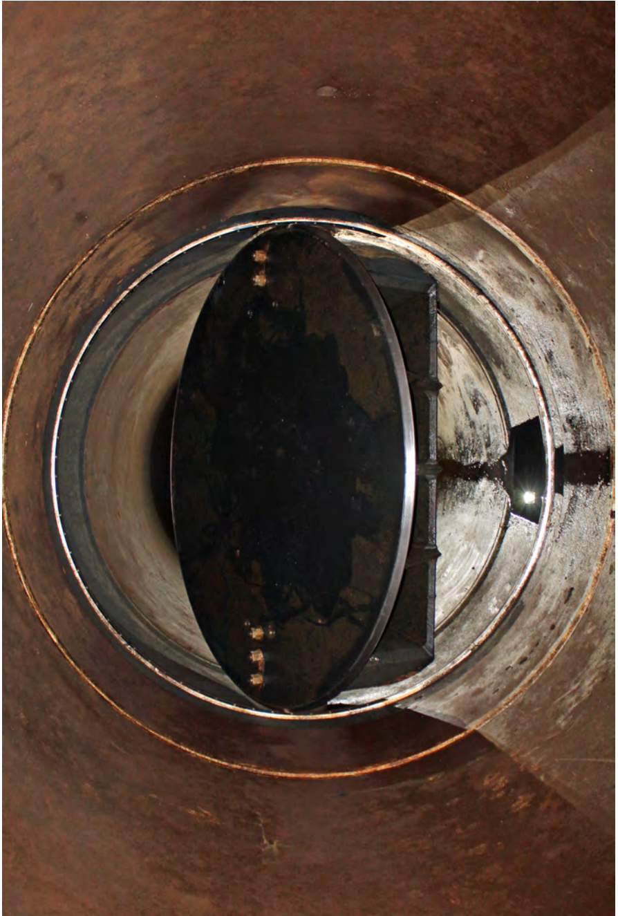
Side view of a 120-inch butterfly valve on the Rialto Feeder.
