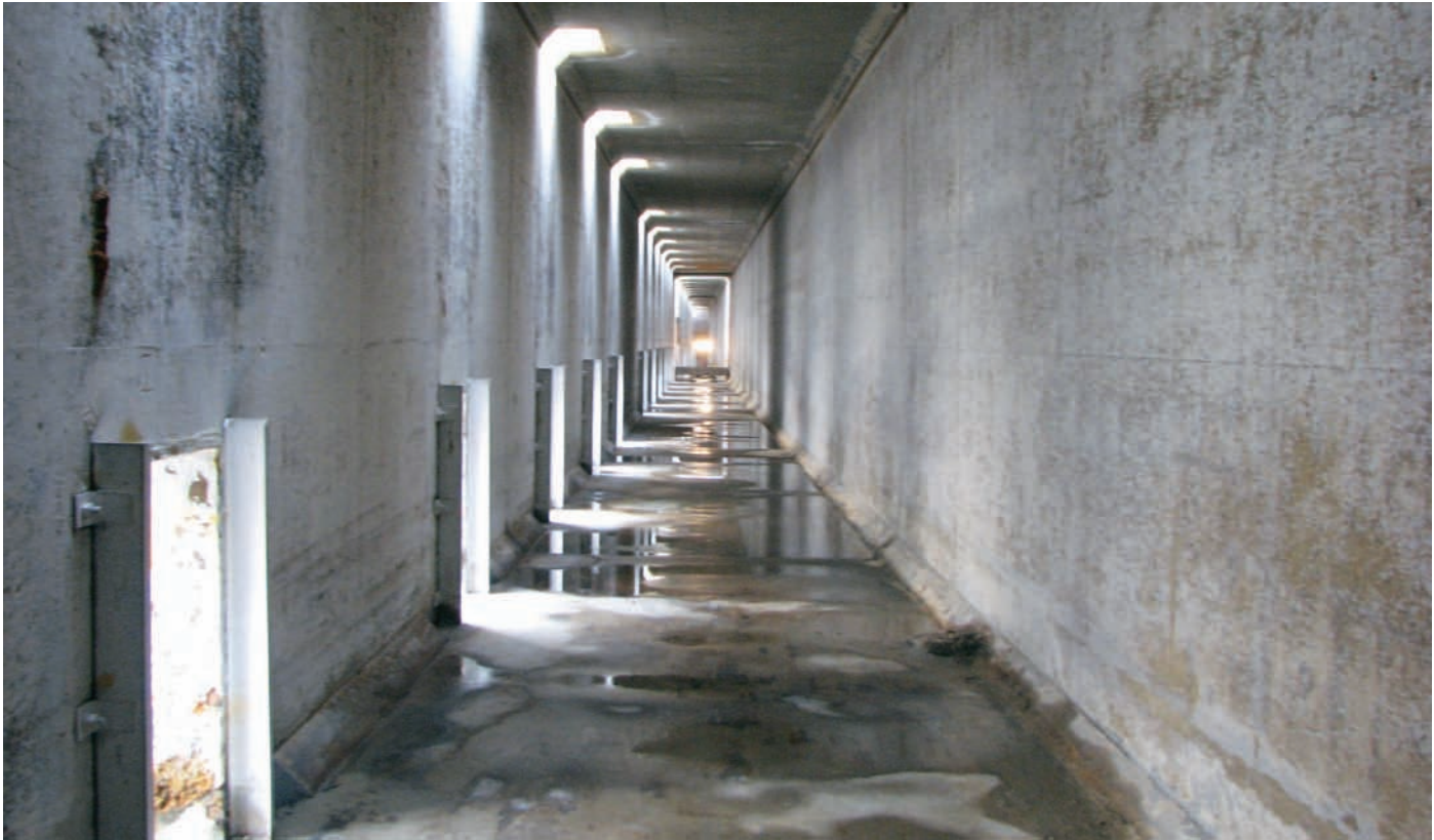
An influent channel at a Metropolitan water treatment plant.
