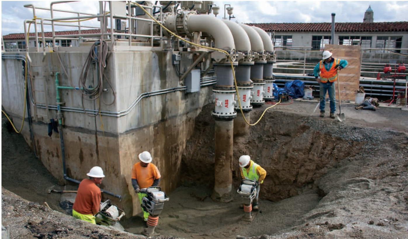
Workers perform a backfilling operation during the Weymouth Water Treatment Plant shutdown.
