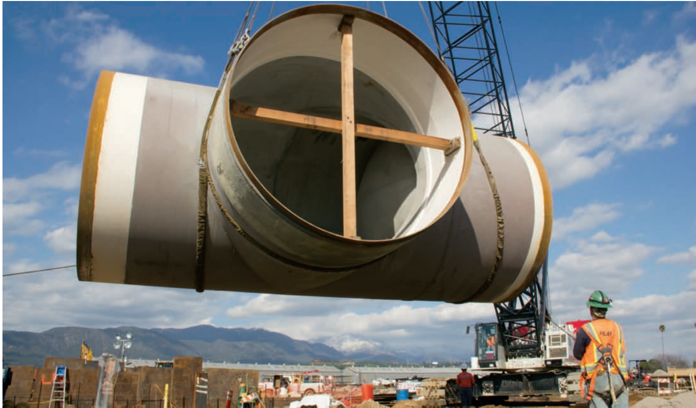
An influent tee is lowered by crane to tie into a newly-installed influent conduit during a treatment plant shutdown.
