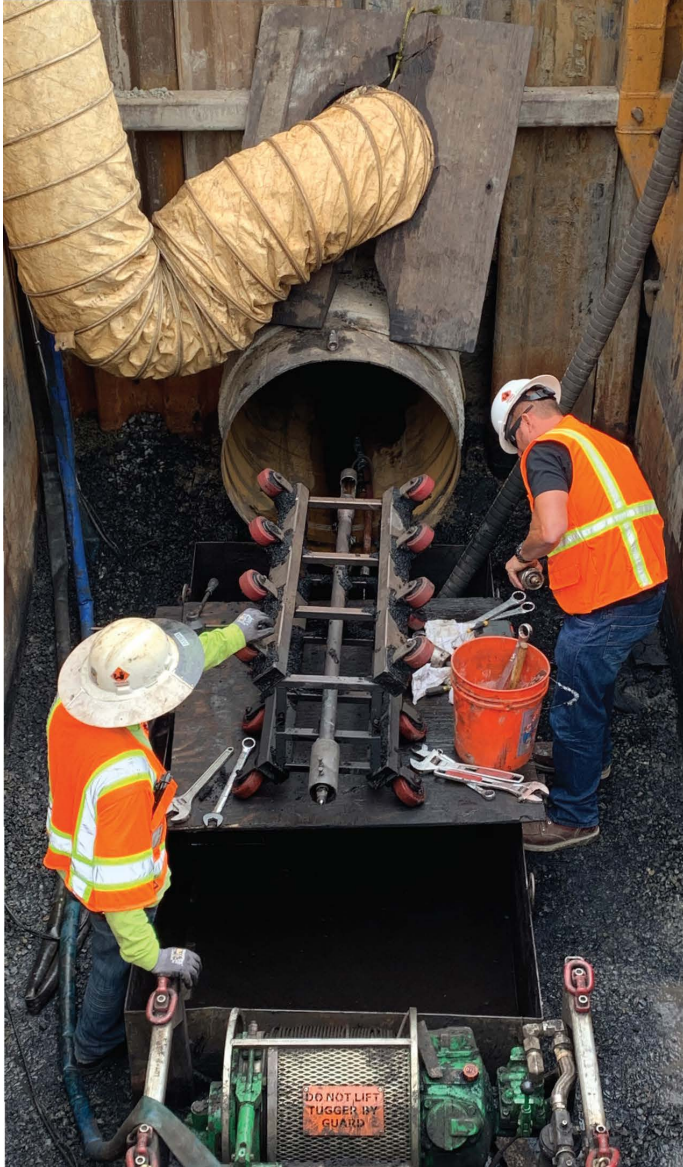
Repair crews extract machine used for removing coal tar lining from the interior of Orange County Feeder, July 2019.
