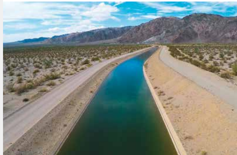
Photo: CRA canal section approaching Hinds Pumping Plant
