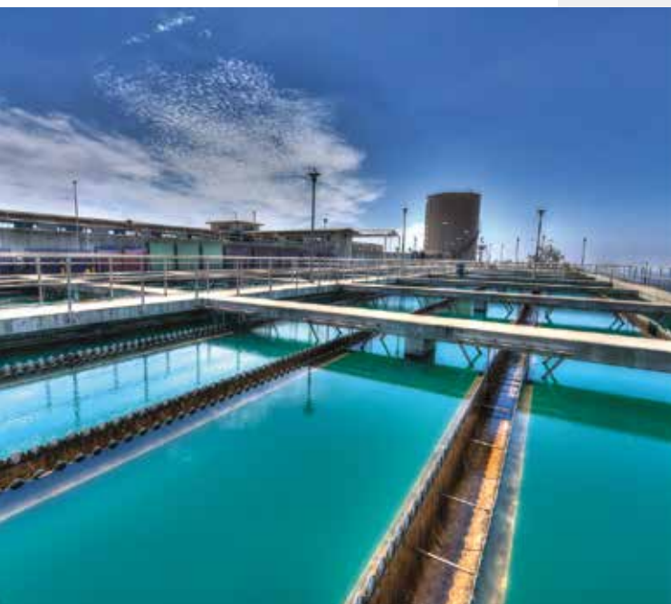
Photo: Diemer Water Treatment Plant
