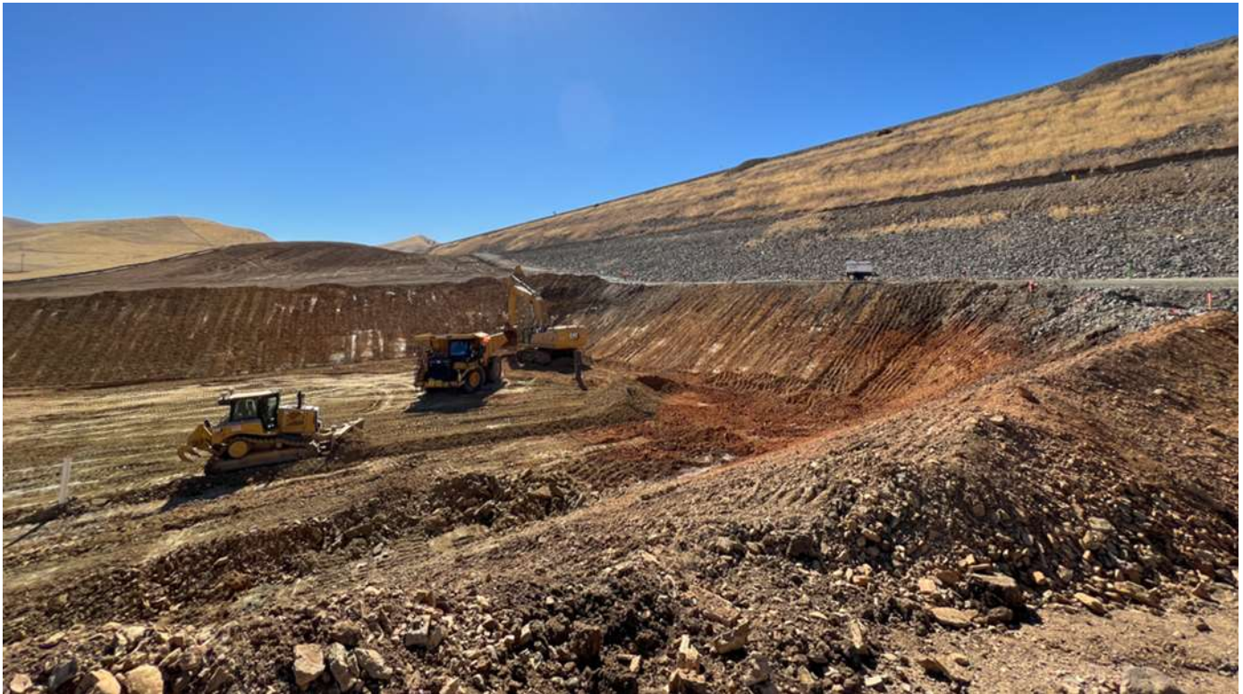
Heavy machinery excavates slope wash material from the base of B. F. Sisk Dam (Photo credit: Reclamation).
