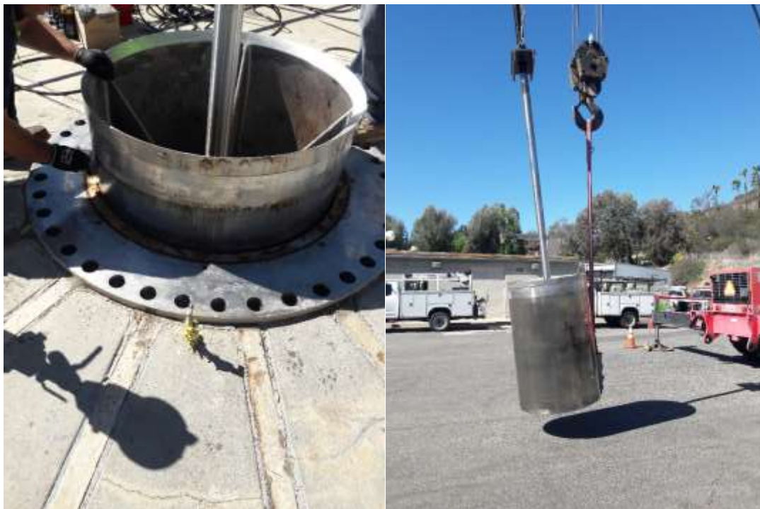
Removal of sleeve valve (left) and valve body (right) at Red Mountain PCS
