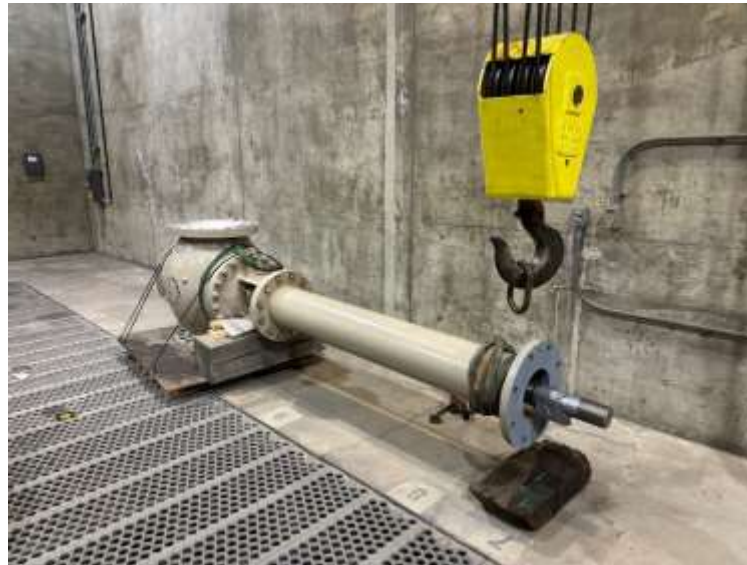
Refurbished motor-operated globe valve for Carbon Creek PCS
