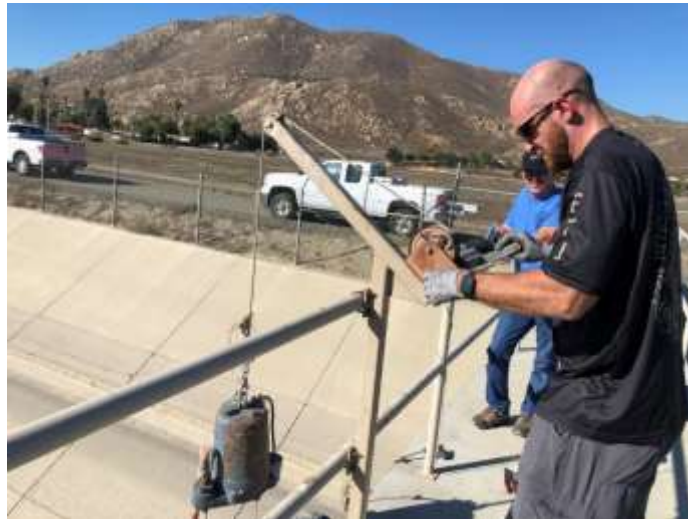
Staff modifying a submersible pump for the San Diego Canal online water quality analyzers
