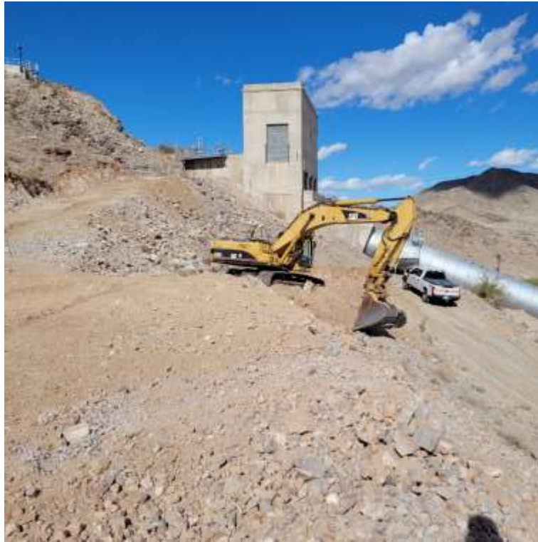
Heavy equipment operators maintain access to the head gate structure at Iron Mountain pumping plant
