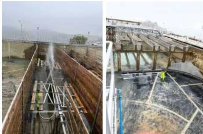
Staff cleaning the basin flocculators (left) and the basin clarifiers (right) at the Diemer plant
