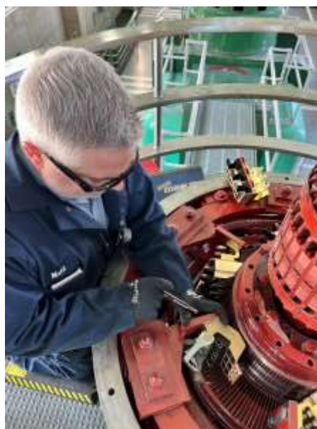
Staff replacing pump brushes at Eagle Mountain pumping plant
