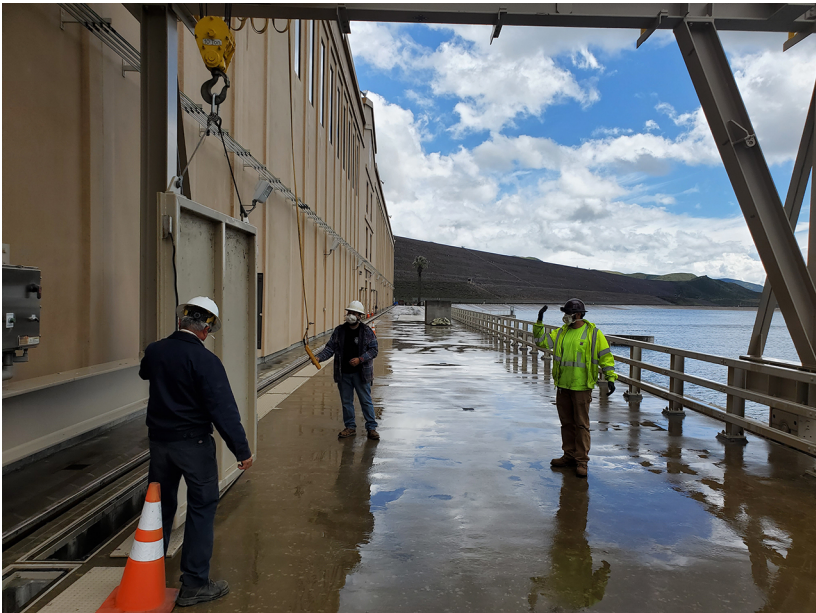
Staff removing an isolation gate at Wadsworth Pumping Plant while adhering to COVID-19 response protocols.
