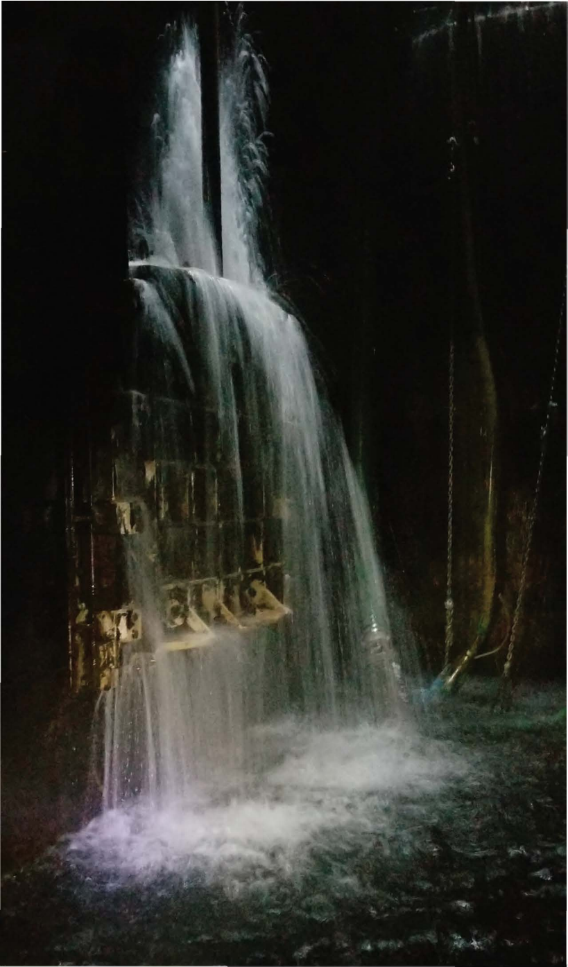
This deceptively beautiful scene shows a leaking slide gate repaired during Metropolitan's 2019/20 shutdown season, which continued even amid the COVID-19 pandemic.
