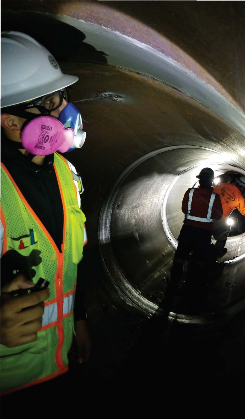
Amid a global pandemic, Metropolitan continued essential work under careful guidelines, including cement mortar lining at Reach 2 of the Second Lower Feeder, April 2020.
