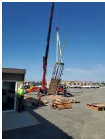
Staff performing test lift of the gate assembly (left) and lowering equipment (right) into the Lake Mathews Forebay
