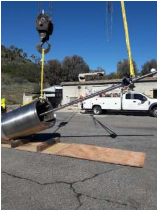
Rigging of valve gate (left) and sleeve valve installation (right) at Red Mountain PCS
