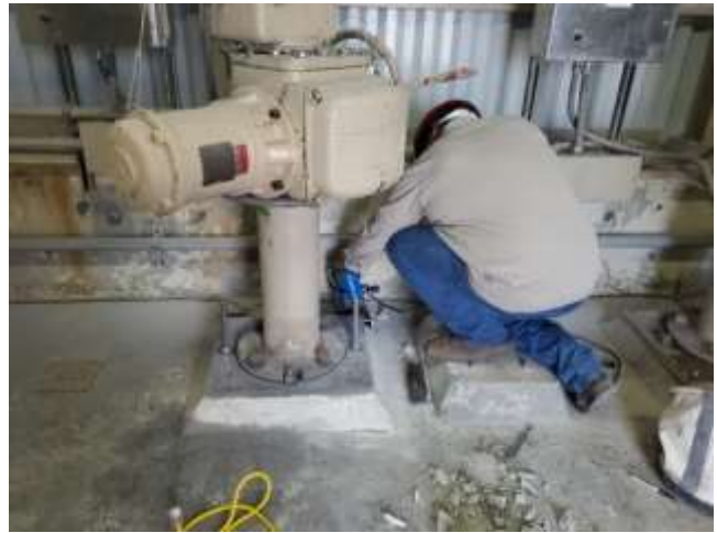
Gate No. 12 with repairs (left) and staff installing additional fasteners to the actuator mounting plate (right) at Lake Mathews
