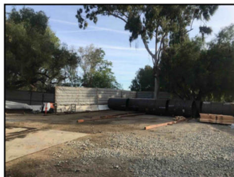
PCCP Second Lower Feeder Reach 3A Noise Barriers at Palos Verdes North Storage Area
