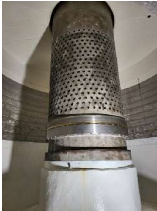
Rigging of valve gate (left) and sleeve valve installation (right) at Red Mountain PCS
