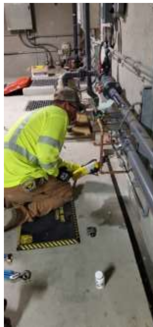
Staff installing backflow prevention device on sodium hypochlorite trench sump pump seal water supply line at the Skinner plant
