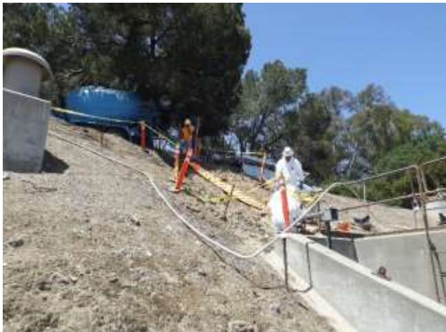
Staff encasing new electric duct bank with concrete (left) and installing new conduit on the lower structure (right) at the Palos Verdes Reservoir
