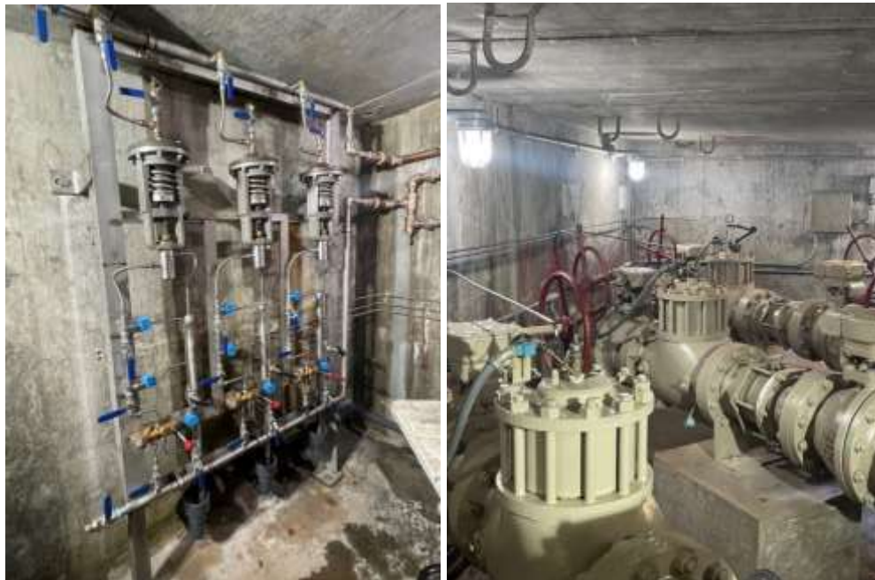
Refurbished pilot valve system on the Santa Monica Feeder at the Sunset Pressure Relief Structure
