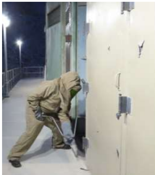
Staff wearing an arc flash suit while racking out 6.9kV electrical circuit breakers
