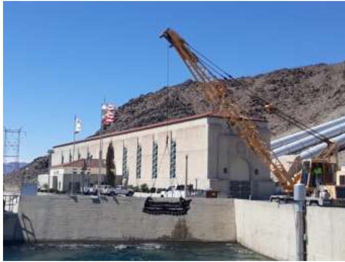
Staff cleaning trash racks at Eagle Mountain pumping plant
