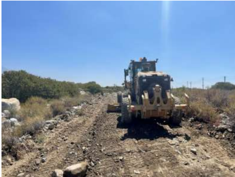
Staff using a motor grader for patrol road repairs along the Rialto Feeder
