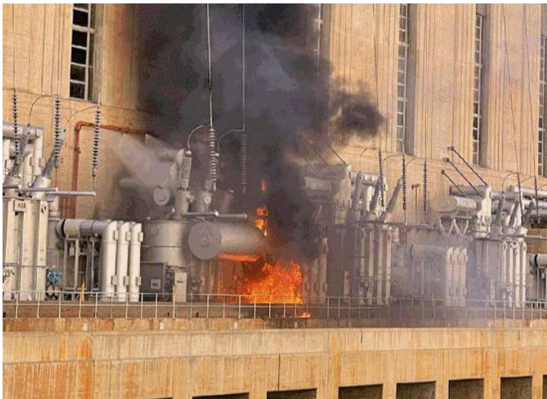
Electrical transformer fire affecting generator units at Hoover Dam ( photo credit: USBR )
