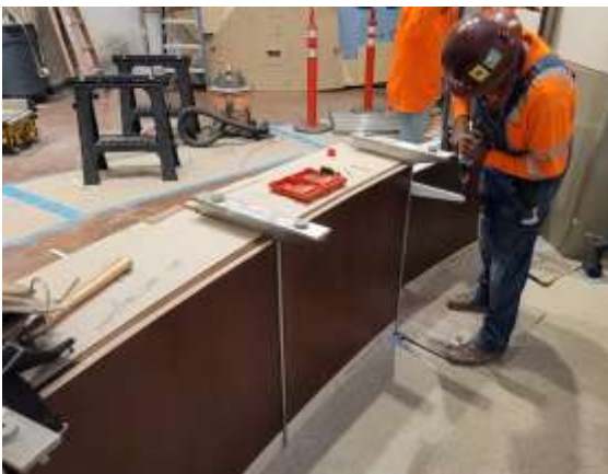
Headquarters Building Improvements —Installing plywood countertop on security desk
