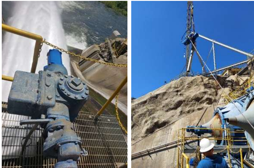
Original actuator in service (left) and new actuator assembly being lowered in place (right) at the San Gabriel Dam
