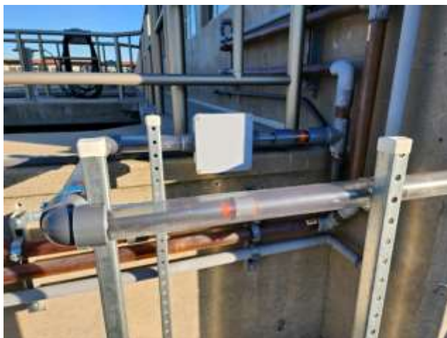
Double containment piping (left) and new containment lance (right) for fluoride injection feed line at the Weymouth plant
