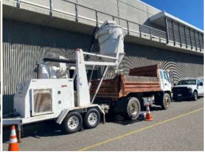
Staff vacuuming quagga mussel shells inside the ozone contactor (left) and using a trailer-mounted vacuum (right) at the Diemer plant
