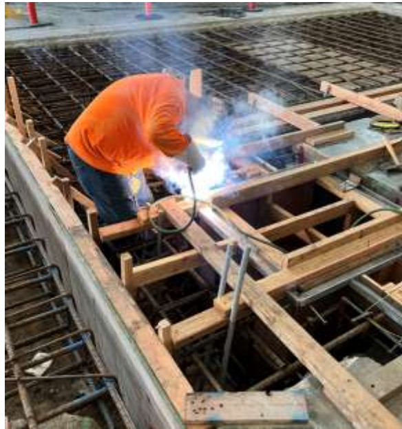
La Verne Shop Improvements—Welding trench drain supports
