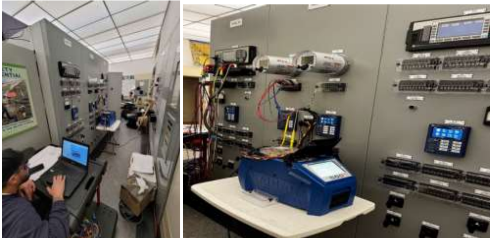
Staff performing system testing on new transformer protection relay panel at Hinds pumping plant
