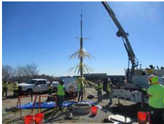
Staff installing pipe-diver device to begin inspection of the Sepulveda Feeder
