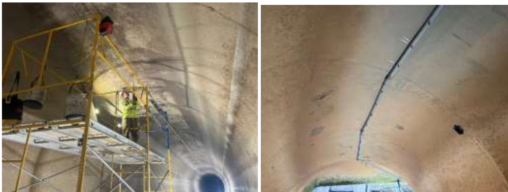
Staff installing conduit (left) and the completed installation (right) along the top of the Hayfield Tunnel
