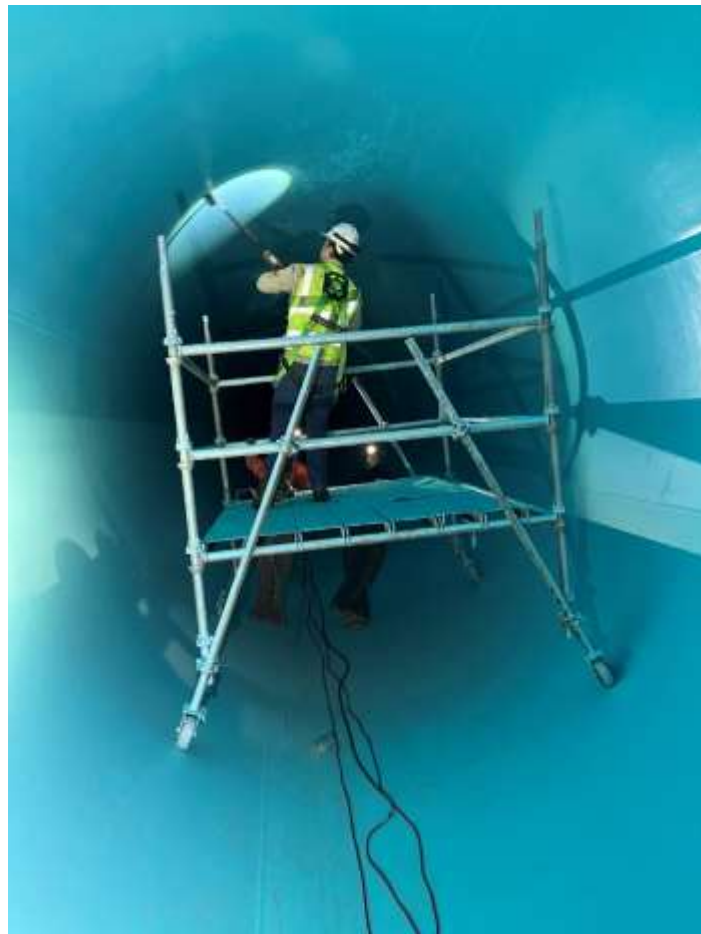
Etiwanda Pipeline Relining—Testing new polyurethane coating
