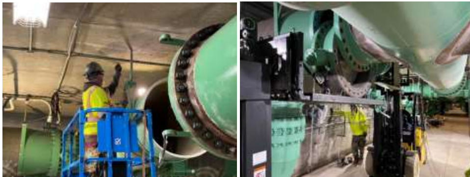
Staff installing lifting points (left) and removing one of two filter valves (right) at the Diemer plant
