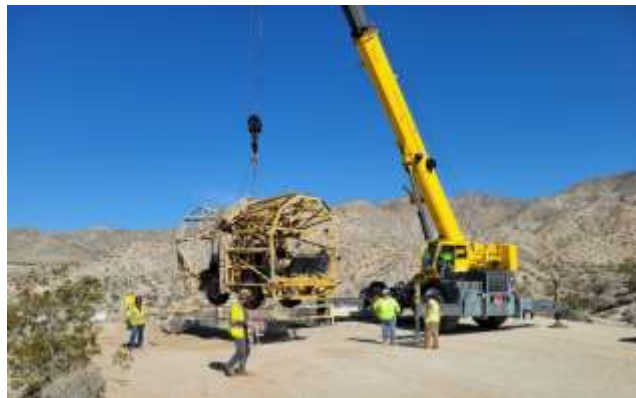
Desert staff lowering the tunnel cleaning machine into the CRA
