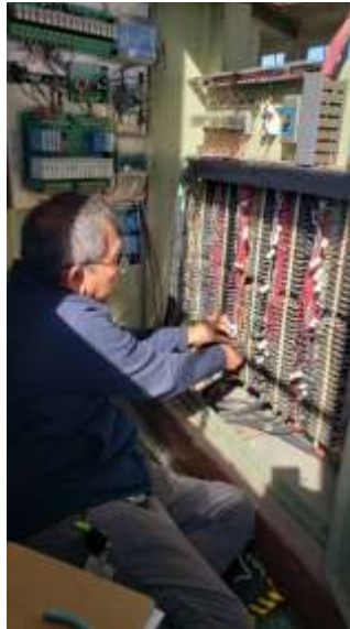
Technician disconnecting power from filter console and labeling conductors
