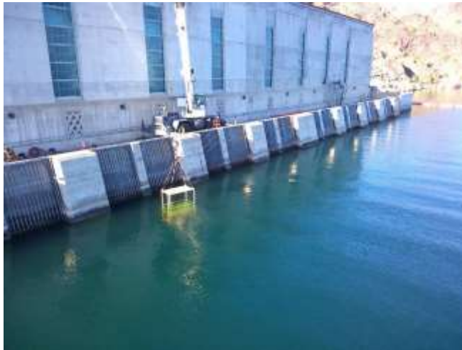
Staff performing maintenance on Intake trash racks
