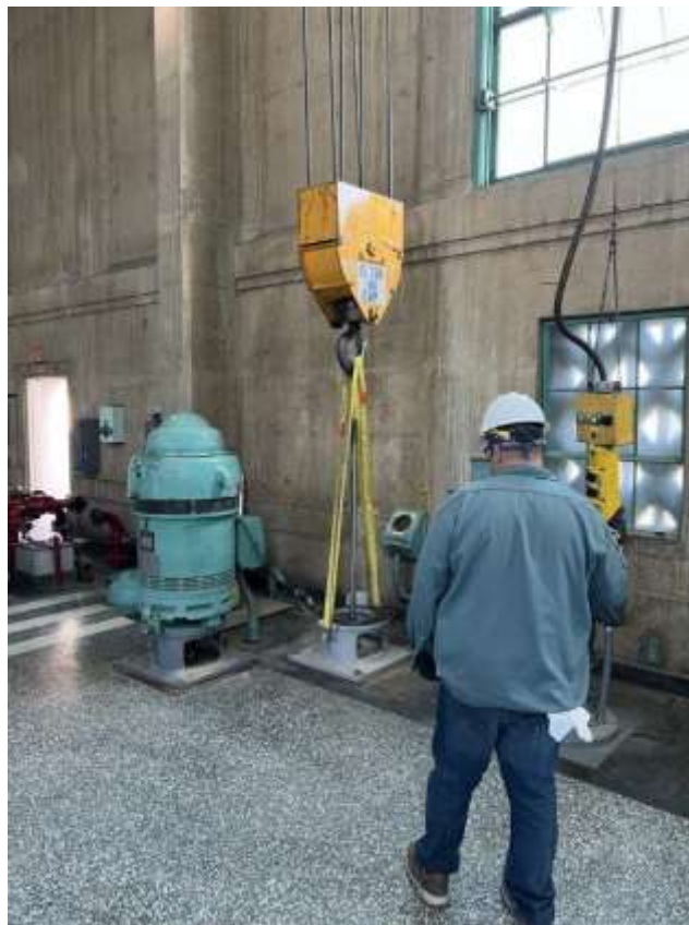
Staff removing a circulating water pump for inspection and repair
