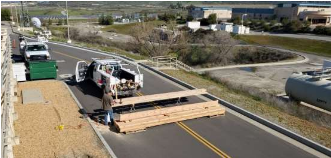
Staff cutting new flocculator baffle boards before installation at the Skinner plant
