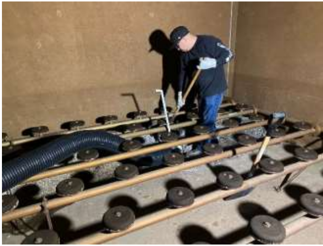
Staff vacuuming quagga mussel shells inside the ozone contactor (left) and using a trailer-mounted vacuum (right) at the Diemer plant
