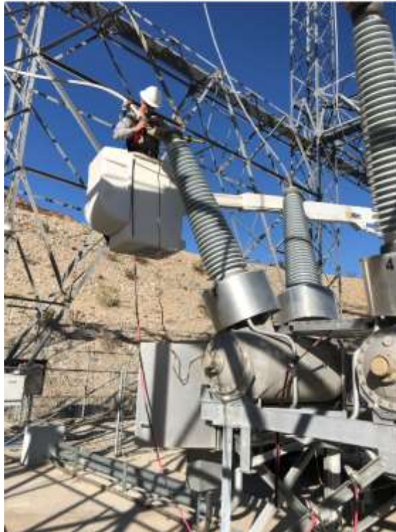
Staff performing maintenance and repairs on a 230kV circuit breaker at Hinds pumping plant
