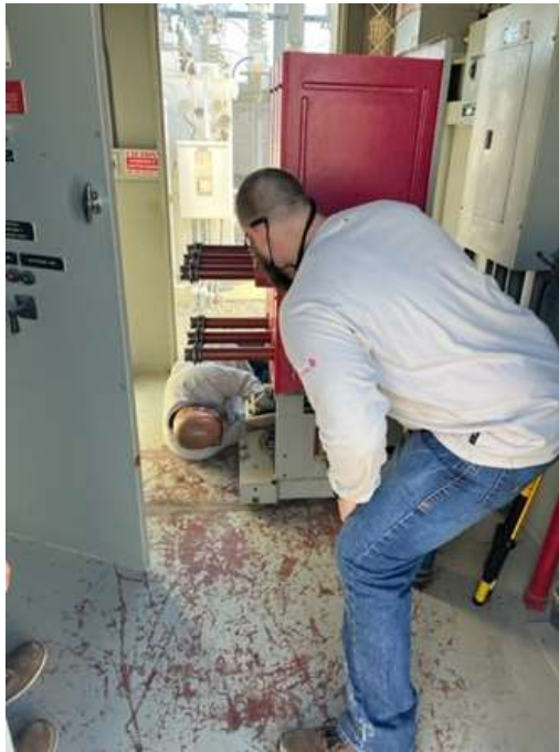
Staff repairing circuit breaker at Temescal HEP
