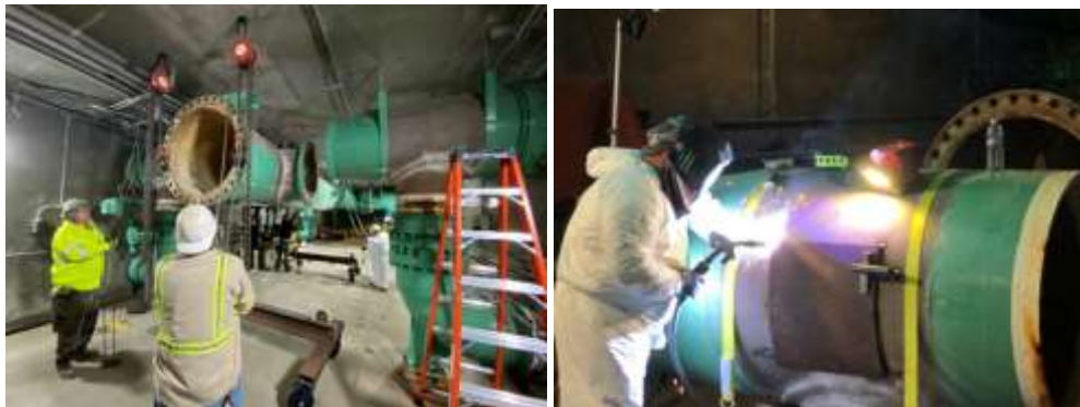
Staff lowering the main backwash line (left) and performing welding repairs (right) at the Diemer plant
