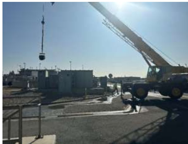
Crane lifting circuit breaker at the Weymouth plant
