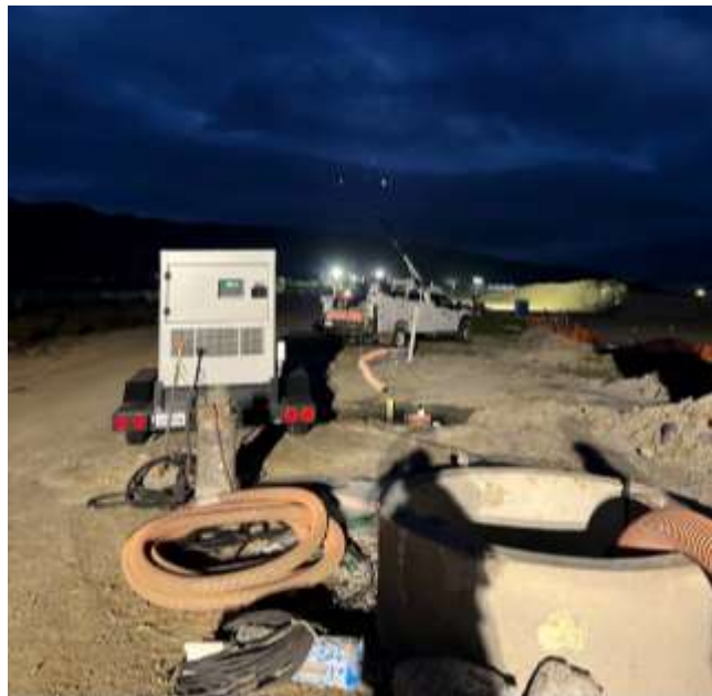
Staff dewatering the Casa Loma Siphon during the CRA shutdown
