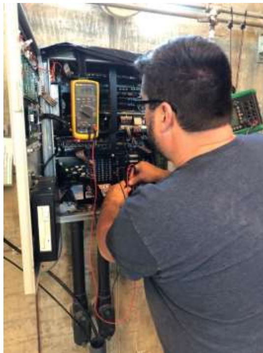
Staff repairing the finished water reservoir influent flowmeter at the Skinner plant
