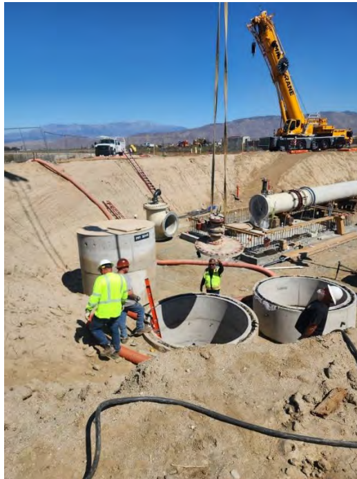
Staff removing flanges during dewatering process of the Inland Feeder
