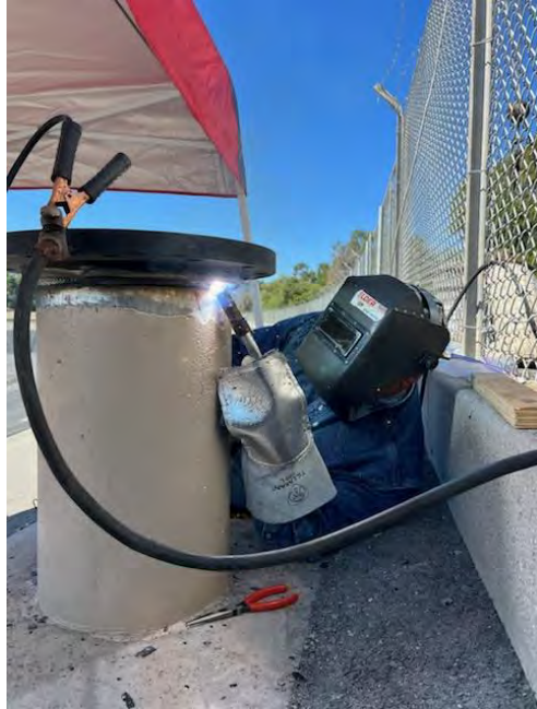
Staff welding flange to the relief piping at Palos Verdes
