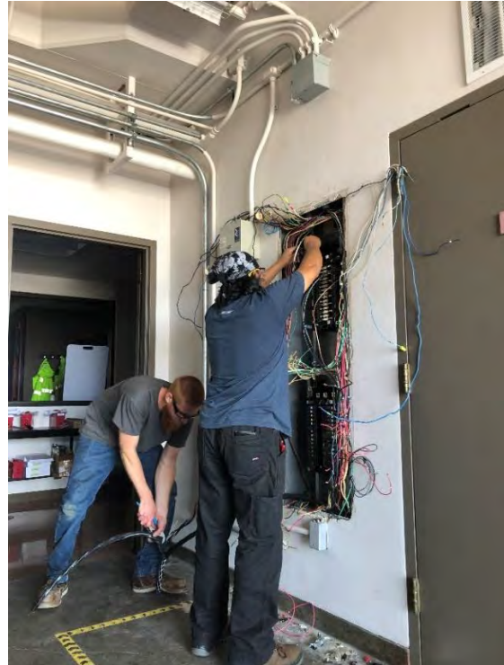
Staff replacing outdated electrical panel at Diemer plant
