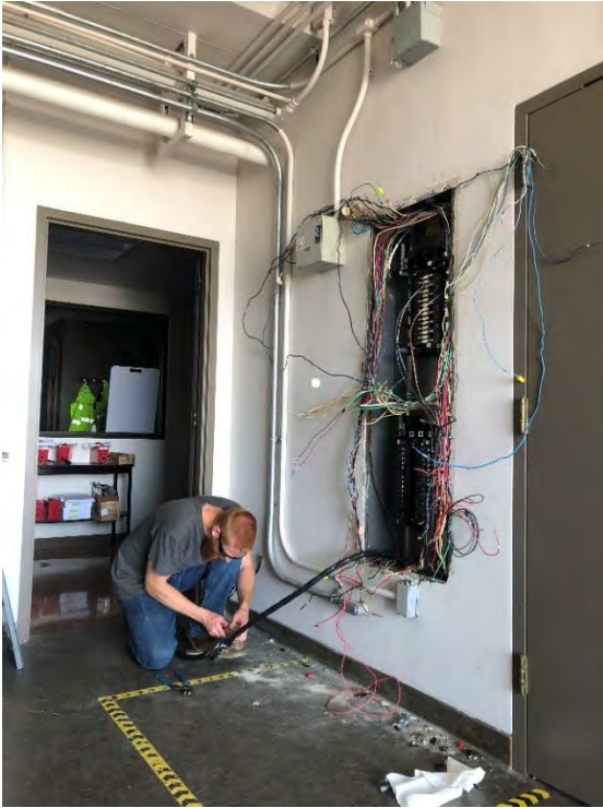
Staff replacing outdated electrical panel at Diemer plant
