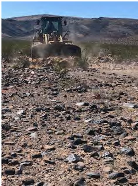
Staff repairs an access road along the 230kV CRA transmission system
