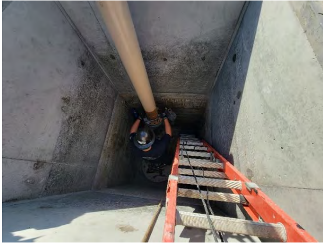
Staff installing blow-off riser (left) and completing structure handrail and cover installation (right)
