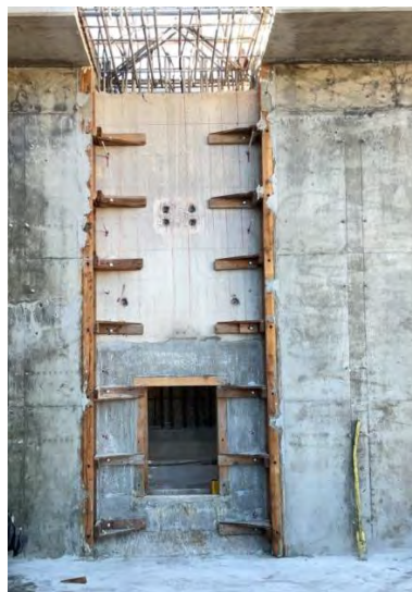
Weymouth Basins 5–8 and Filter Building No. 2 Rehabilitation — Basin 7 slide gate wall overlays
