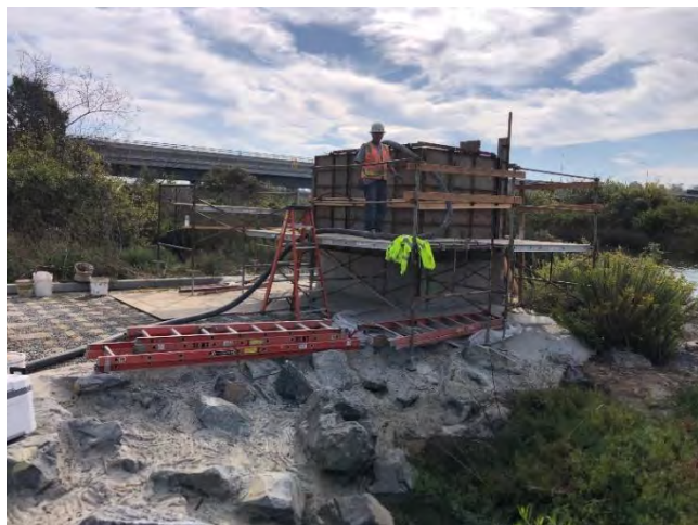
Staff preparing to pump concrete (left) to increase structure height (right)
