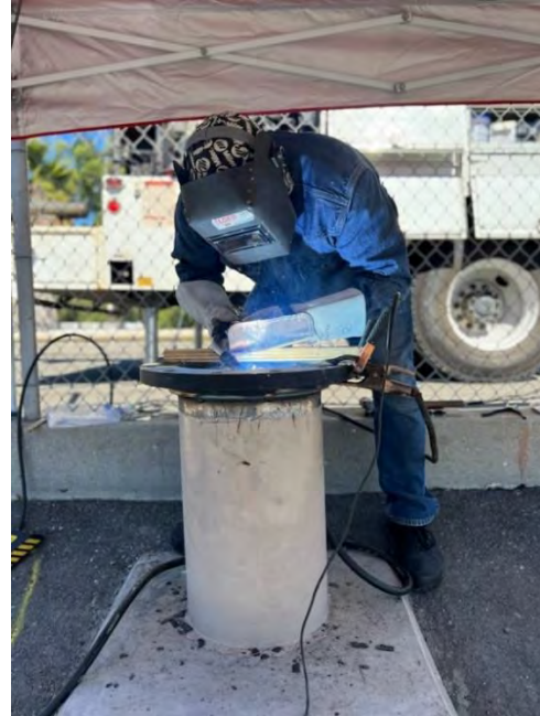
Staff welding flange to the relief piping at Palos Verdes
