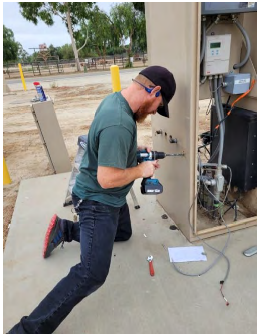
Staff upgrading RTU enclosure used for relaying distribution system flow data
