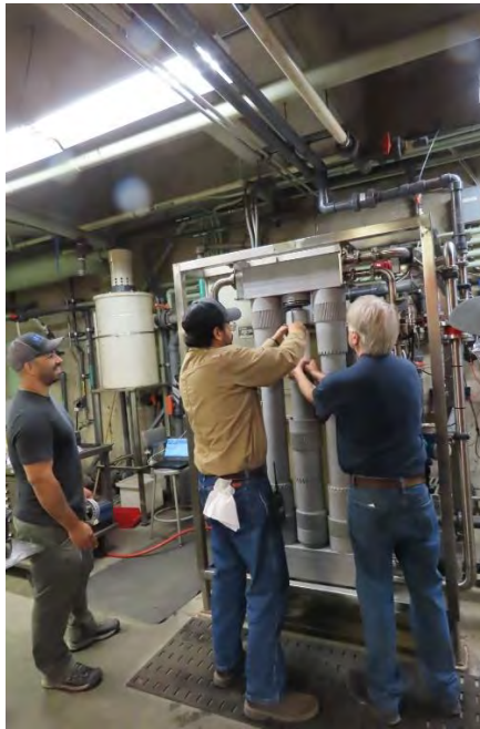
Staff replaces membranes for the domestic water system at a CRA pumping plant
