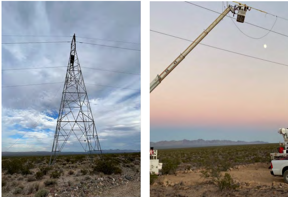
Broken static line (left) and staff splicing the static line (right) on the 230kV CRA transmission system
