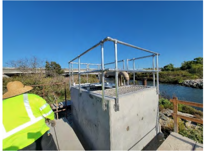
Staff installing blow-off riser (left) and completing structure handrail and cover installation (right)
