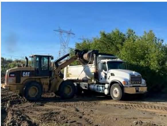
Loader and dump truck loading solids (left) and unloading at the staging area (right)
