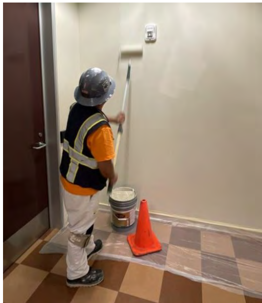
Headquarters Building Fire Alarm and Smoke Control System Upgrades – Restorative painting in Level 1 Elevator area
