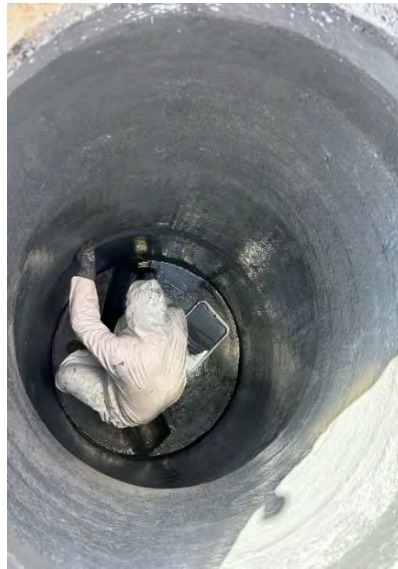
Lake Mathews Wastewater Replacement— Interior coating prep in wastewater access-hole at new Valve Storage Building
