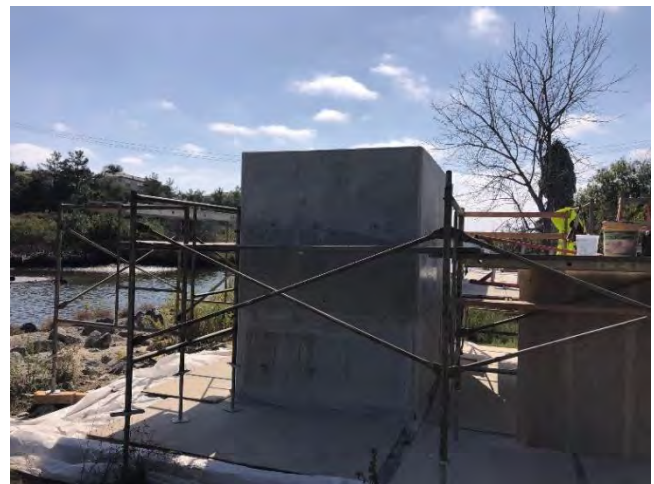
Staff preparing to pump concrete (left) to increase structure height (right)
