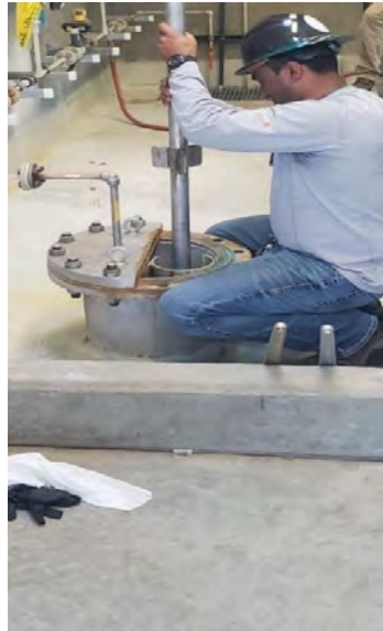
Staff installing non-corrosive FSA injection diffuser for the Skinner FWR
