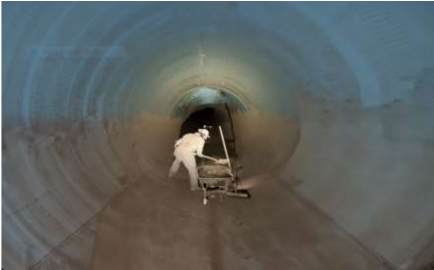
Etiwanda Pipeline Relining—Clean up
