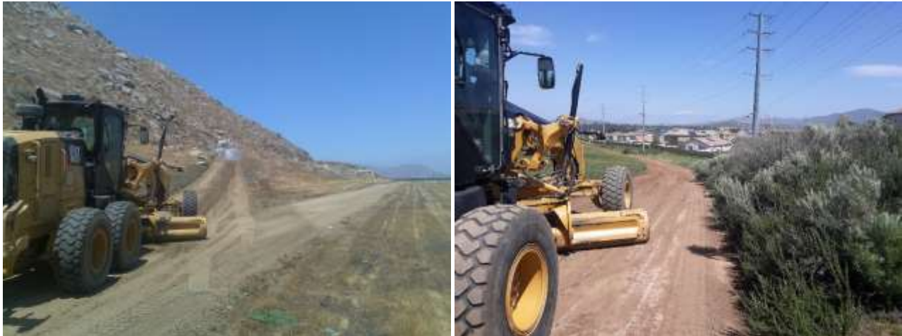
Motor grader and water truck performing routine maintenance along the CRA (left) and San Diego Canal (right) patrol roads
