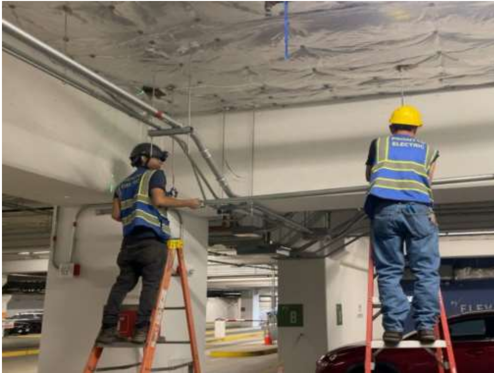
Headquarters Building Fire Alarm and Smoke Control System Upgrades —Level P1 conduit installation
