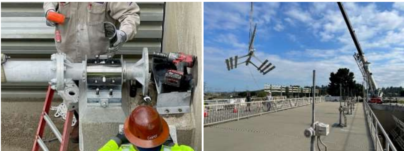
Staff disassembling wet side pillow block (left), and crane operators hoisting flocculation shafts (right) at the Jensen plant
