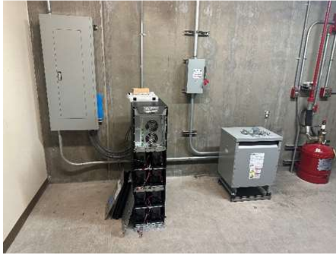
UPS and electrical equipment ready for start-up at the Weymouth plant
