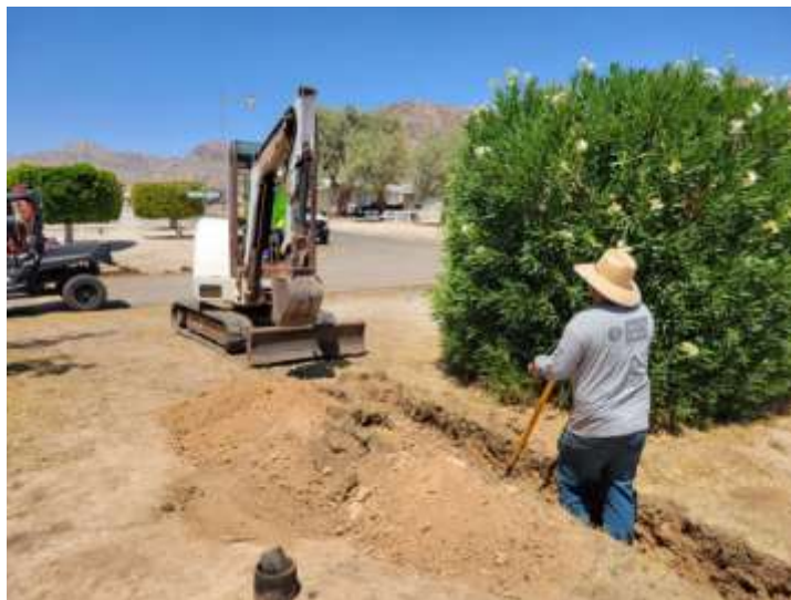
Staff excavating to replace an aging sewer line at the Iron Mountain pumping plant
