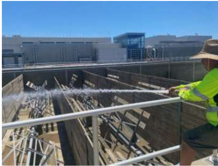
Staff washing down the sedimentation basin at the Diemer plant
