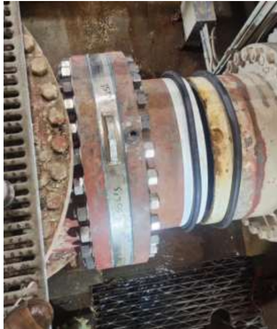
The multi-orifice plate installed into the 30-inch line at Covina PCS
