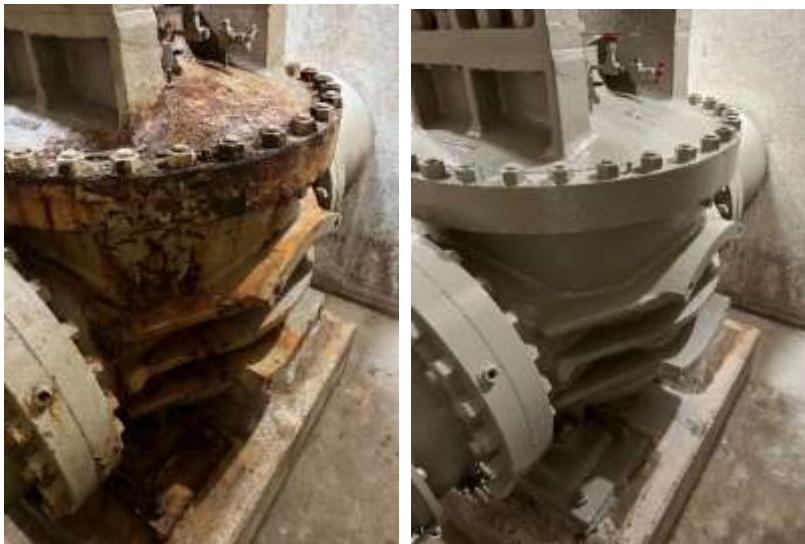
Before (left) and after (right) coating work on a plug valve at the PM-24 service connection
