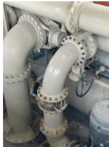
Survey report of the existing elbow (left), fabrication of new elbow (middle), and installed new elbow (right) at the Weymouth plant
