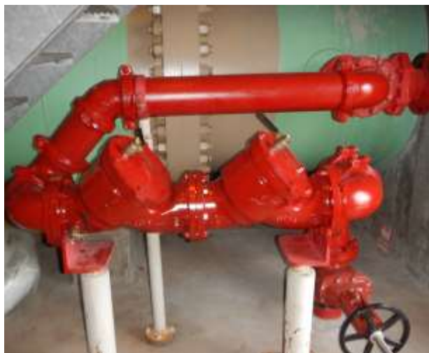
OC-88 Fire Sprinkler—New backflow preventer and piping
