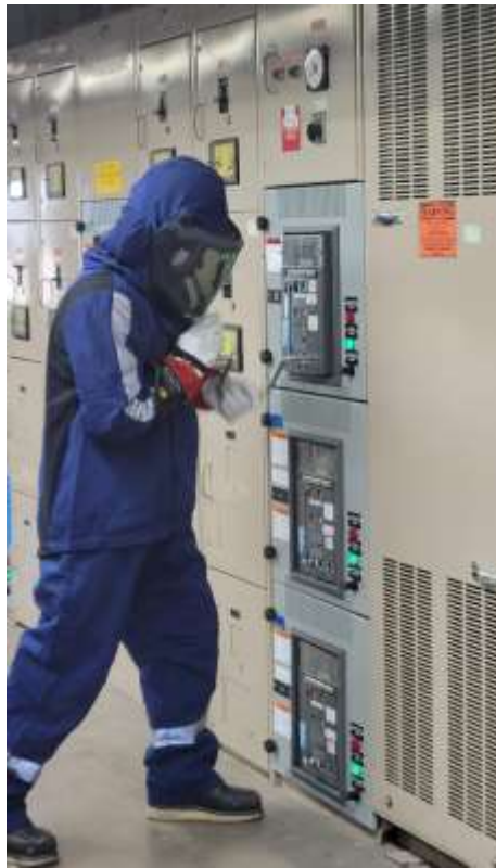
Staff safely racking out 4,160v breaker for maintenance at the Mills plant
