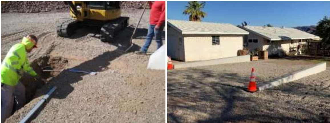
Staff excavating around buried utilities (left) and finished canopy footings (right) at a Desert facility residential structure
