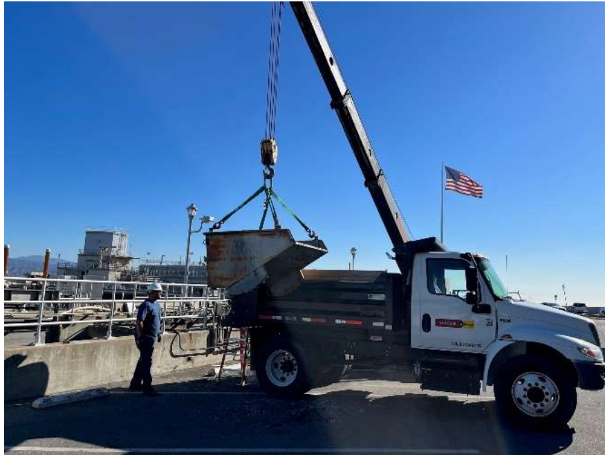
Staff removing solids and quagga mussel shells during maintenance of the basin influent channel at the Diemer plant
