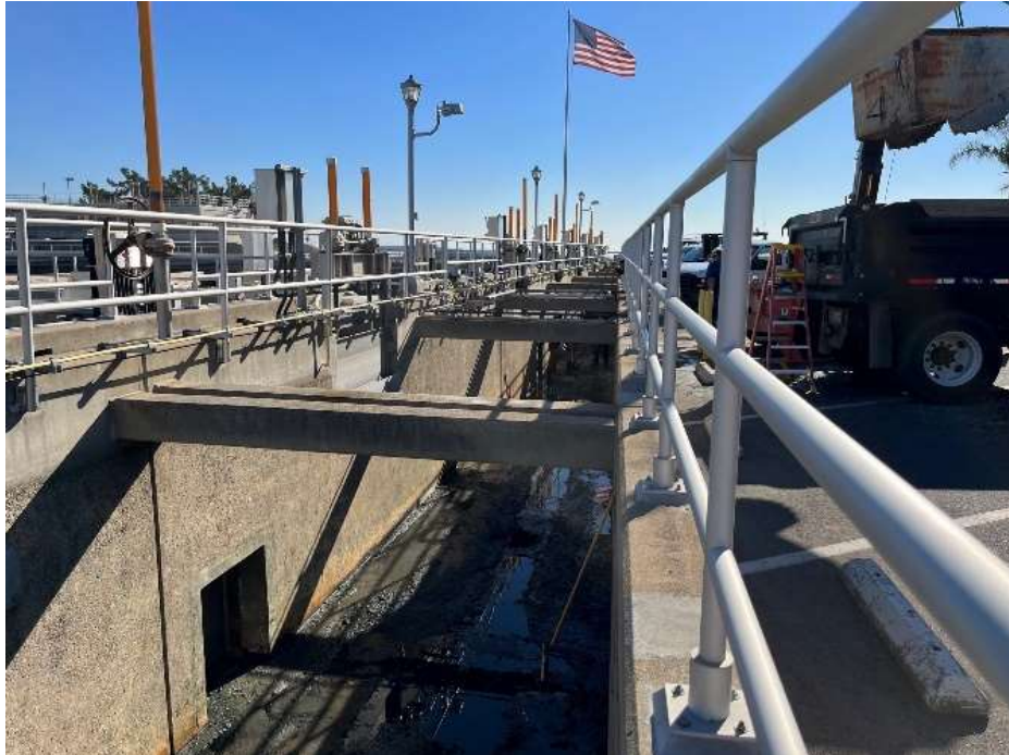
Basin influent channel at the Diemer plant
