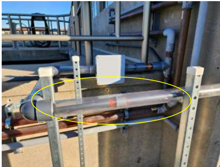
Double containment piping for the fluoride injection system at the Weymouth plant
