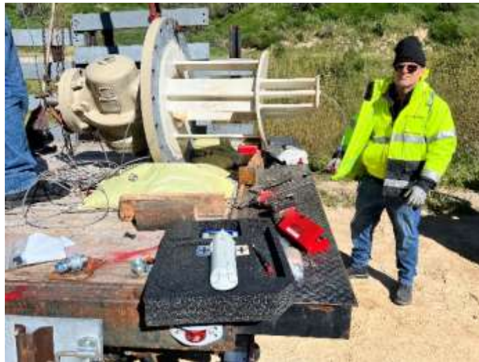
Staff repairing the LADWP service connection flow meter at Magazine Canyon
