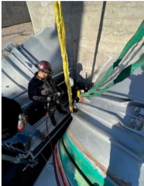
Staff installing a discharge line isolator at Iron Mountain pumping plant
