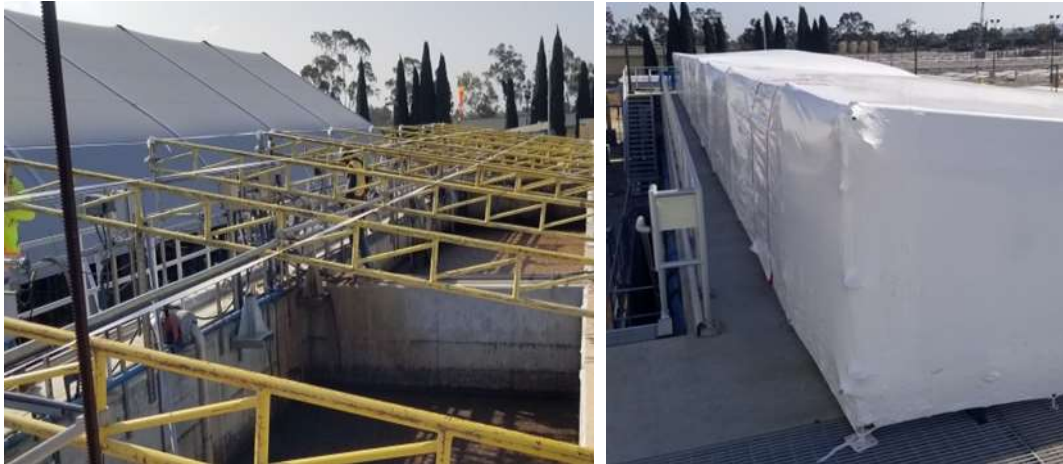
Installation of an enclosure over bioreactors to support SCAQMD air permit source testing at the demonstration plant
