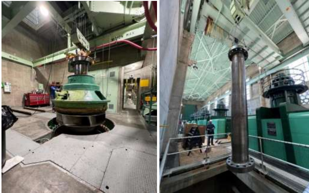
Staff removing the pump (left) and pump shaft (right) of a discharge valve at Iron Mountain pumping plant
