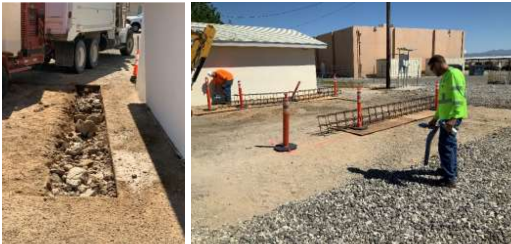
Vacuum excavation revealing rock (left) and staff locating buried utility conflicts (right) at a Desert facility
