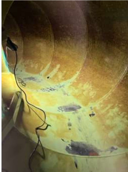
Scroll case prepared for inspection at Lake Mathews HEP
