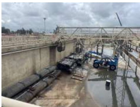
Contractor Removing Internal Components at Basins 7 and 8 for the Weymouth Basins 5–8 Rehabilitation Project
