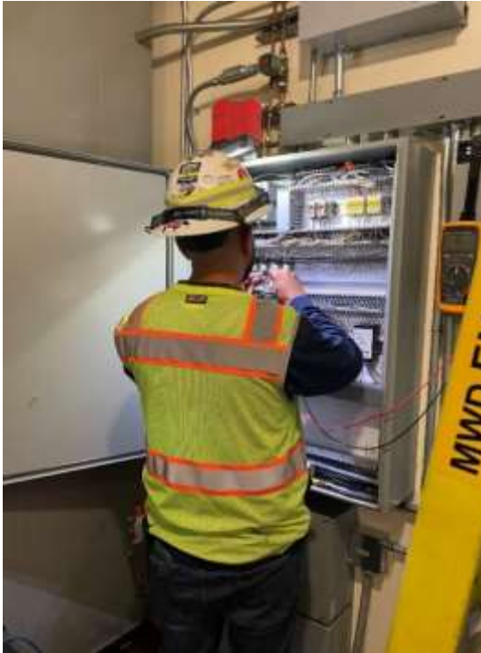
Headquarters Building Fire Alarm and Smoke Control System Upgrades Commissioning smoke and fire detectors
