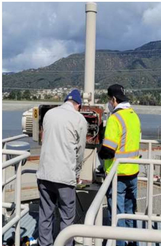
Staff installing new valve position element at Live Oak Reservoir
