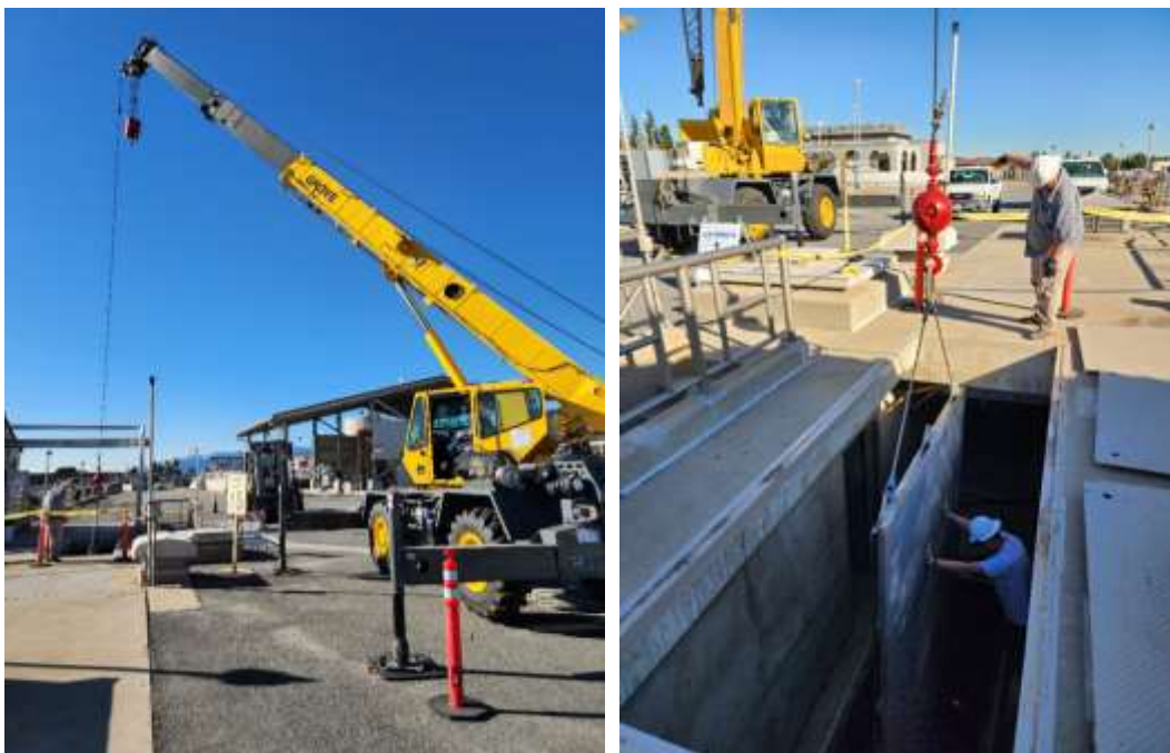
Staff using a crane to lower the isolation gate (left) and guiding the isolation gate (right) into the Effluent Channel at the Weymouth plant
