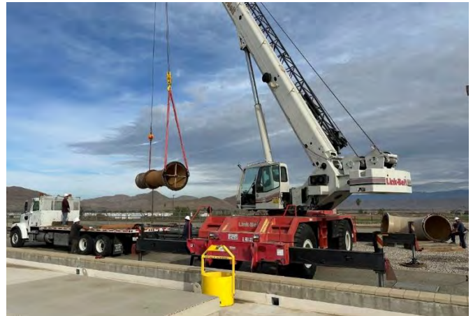
Staff removing six sleeve valves for refurbishment at PC-1
