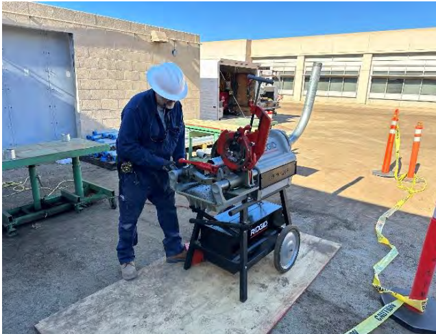
Staff threading electrical conduit (left) and cutting and preparing conduit for installation (right) at the Water Quality Laboratory
