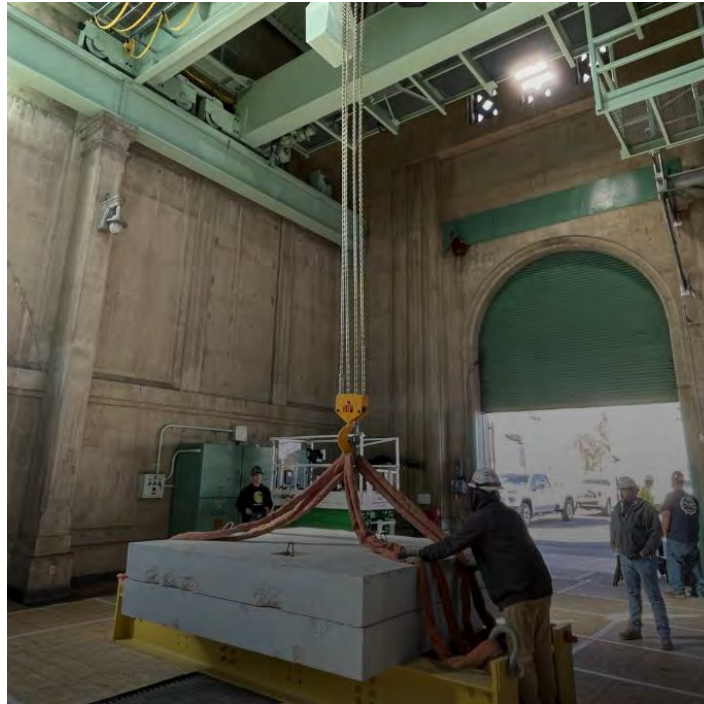
CRA Overhead Cranes Replacement —Eagle Pumping Plant Crane Load Test
