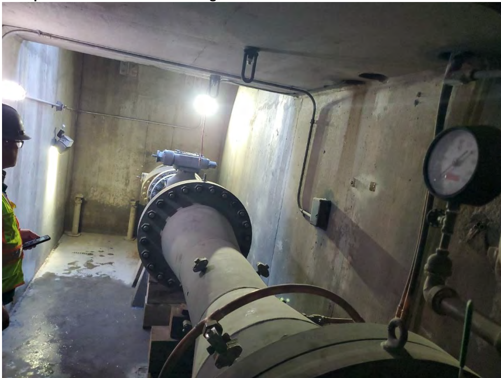
Newly installed venturi flow meter at service connection off the Santa Monica Feeder
