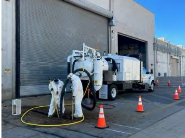
Staff potholing existing utilities (left) and excavating gas line lateral (right)
