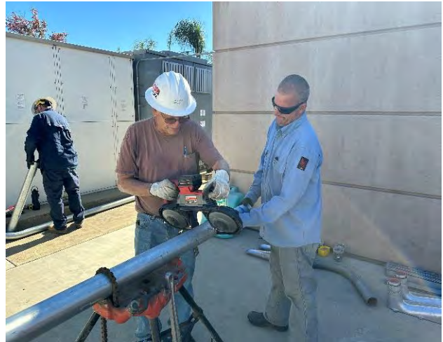
Staff threading electrical conduit (left) and cutting and preparing conduit for installation (right) at the Water Quality Laboratory
