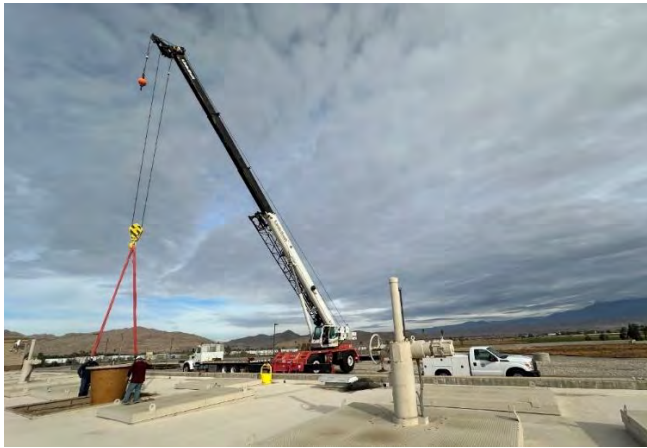
Staff removing six sleeve valves for refurbishment at PC-1
