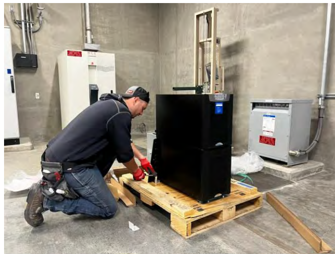
Staff preparing to replace a UPS at the Diemer plant
