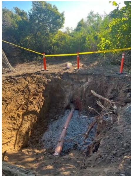
Repaired sewer line at Diemer plant
