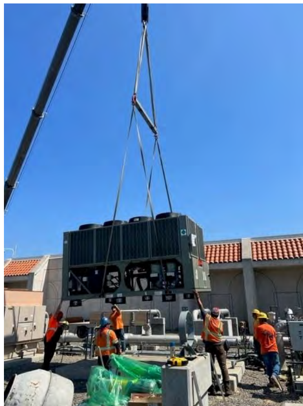
OC-88 Pump Station Chillers Replacement Installation of chiller
