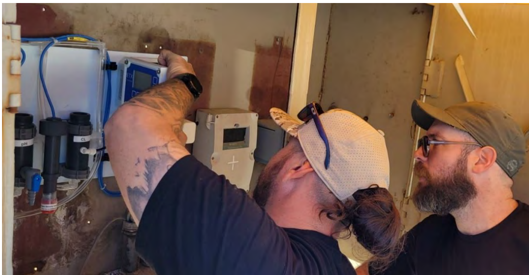
Staff installing chlorine residual analyzer with improved raw water compatibility along the CRA at Cabazon
