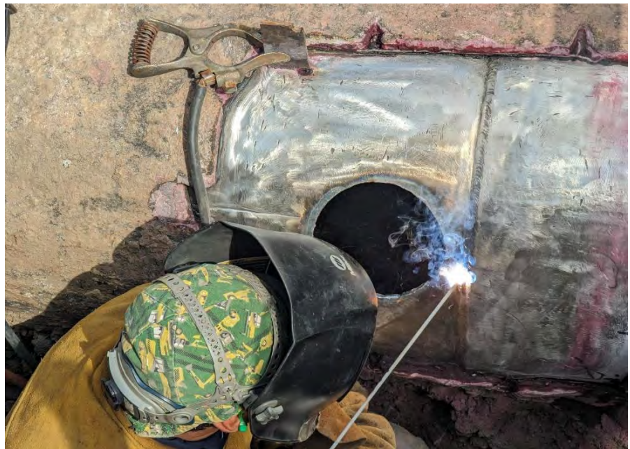
Staff measuring damage area (left) and welding (right) to repair the Compton Lateral
