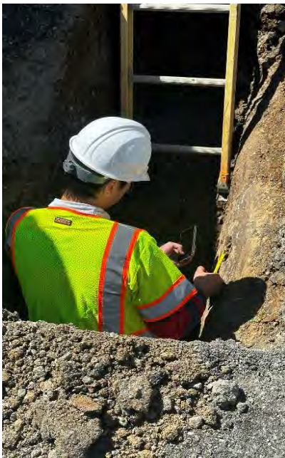
Staff measuring damage area (left) and welding (right) to repair the Compton Lateral
