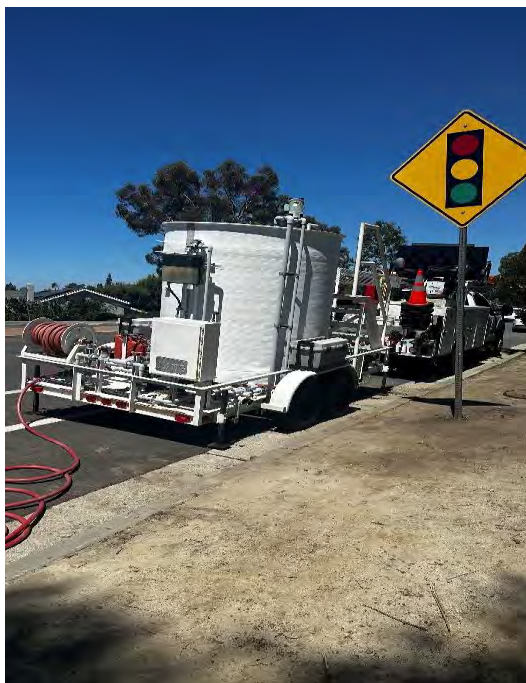
De-chlorination set up at flushing location on Allen McCulloch Pipeline (right) and flushing location on West Coast Feeder (left)
