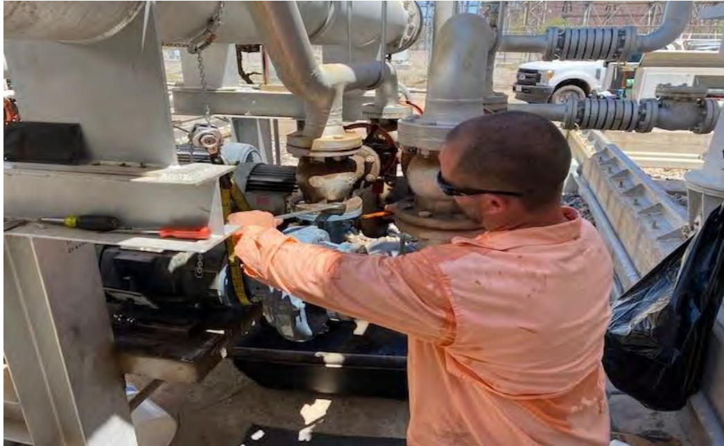
Staff installs a rebuilt forced oil pump on a 230kV transformer along the CRA
