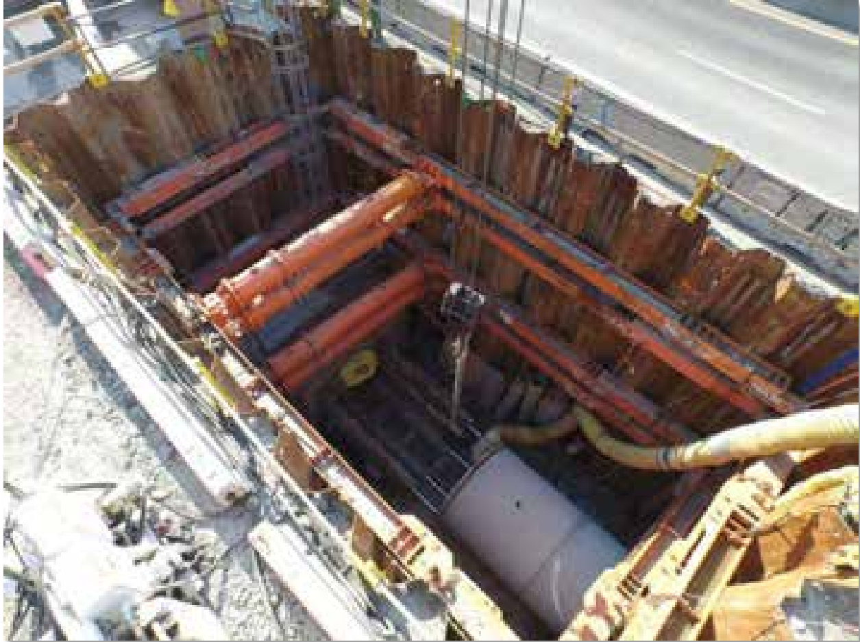
Figure 3-13 Pipe Jacking from a Rectangular Shaft, ConstructionEquipmentGuide.com
