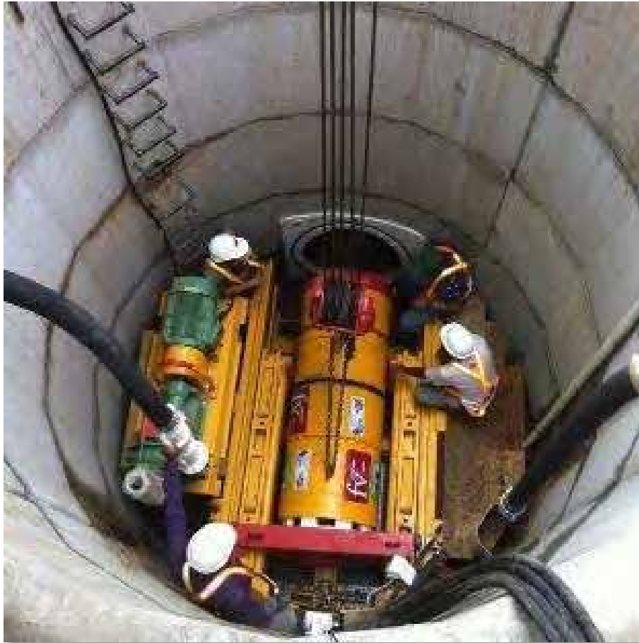
Figure 3-12 Pipe Jacking from a Circular Shaft, Pipe Jacking Association
