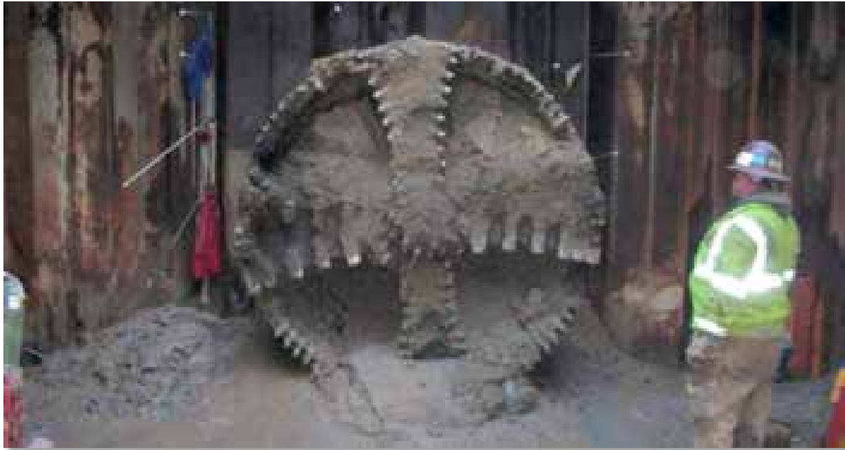
Figure 3-6 72-inch diameter Microtunneling Machine – East Chicago, Indiana
