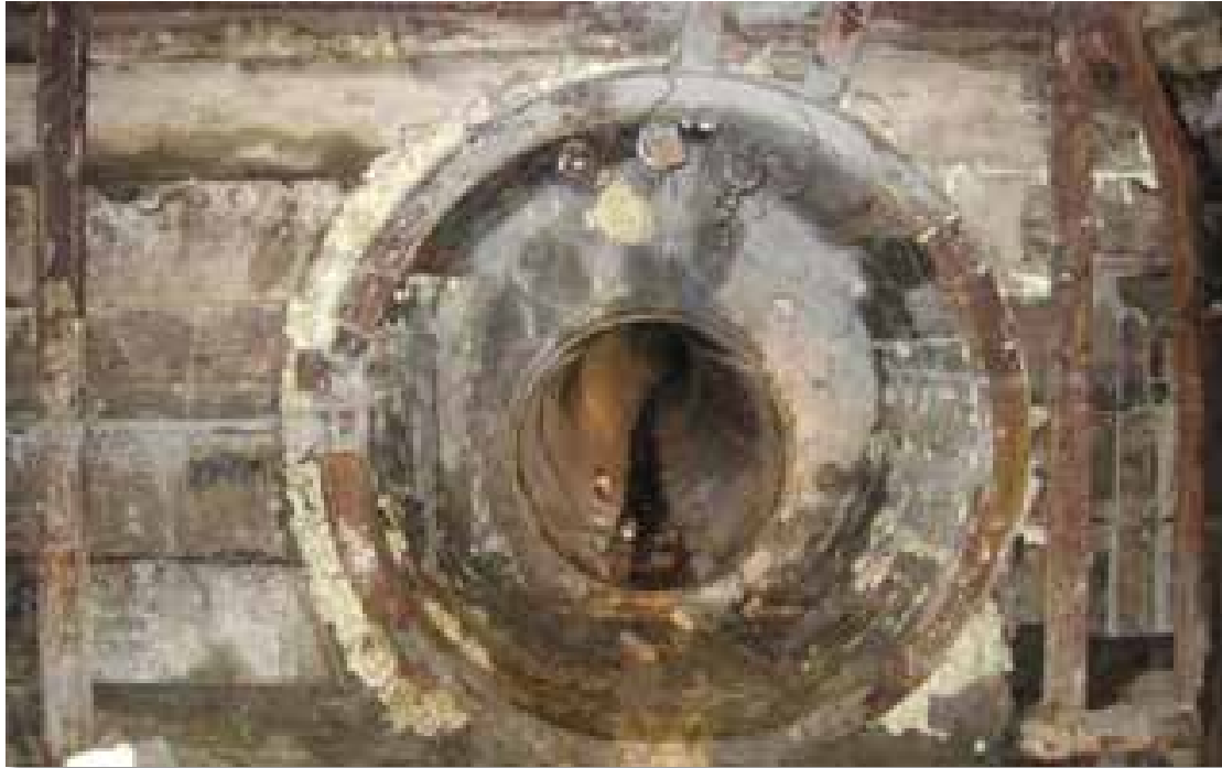
Figure 3-14 Carrier Pipe (Fiberglass) Installed in a Larger Excavated Tunnel, Black & Veatch
