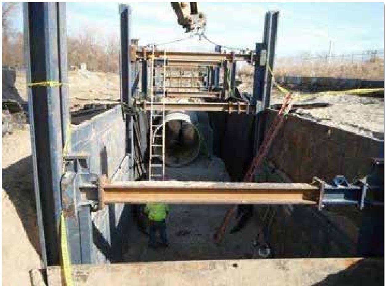
Figure 3-11 Soldier Piles and Steel Plates, Black & Veatch
