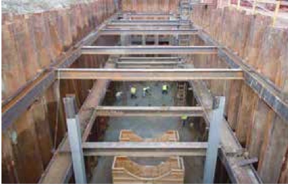
Figure 3-9 Sheet Pile Excavation Support System, Black & Veatch
