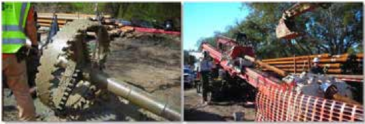
Figure 3-4 Large Diameter HDD Reaming Tool and Drilling Equipment
