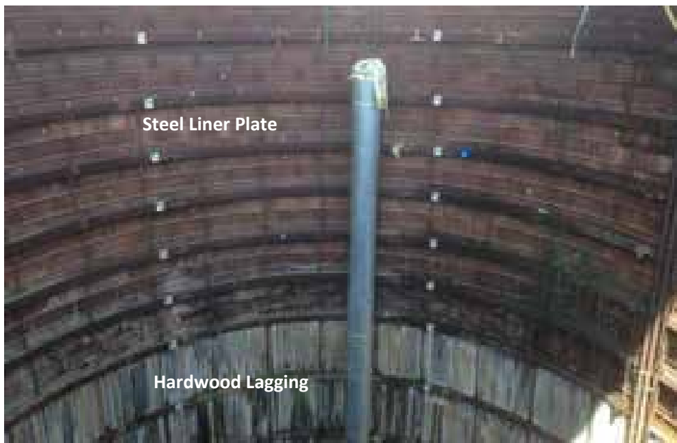
Figure 3-10 Steel Ribs with Steel Liner Plate (Top) and Hardwood Lagging (Bottom), Black & Veatch
