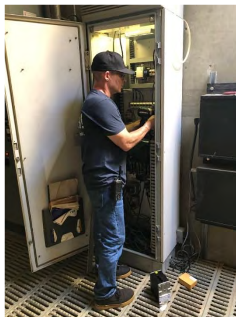
Skinner staff replacing distribution system network switch in Auld Valley PCS
