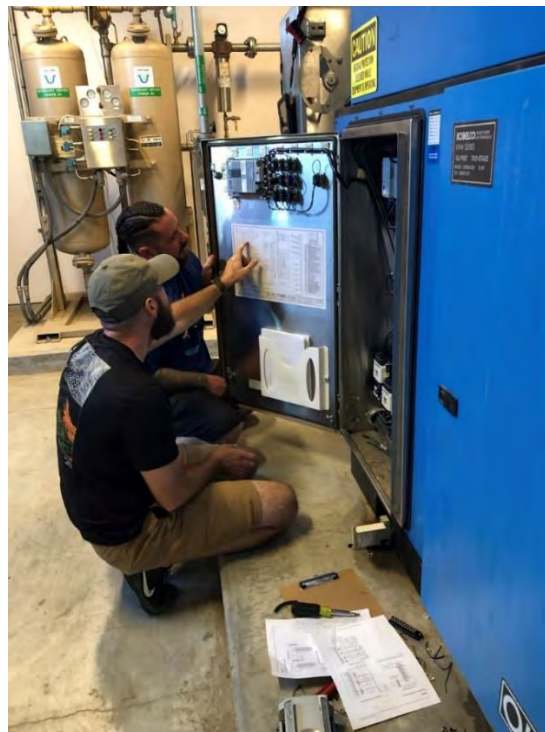
Staff troubleshooting and preparing to upgrade ozone contactor maintenance air compressor PLC at the Skinner plant
