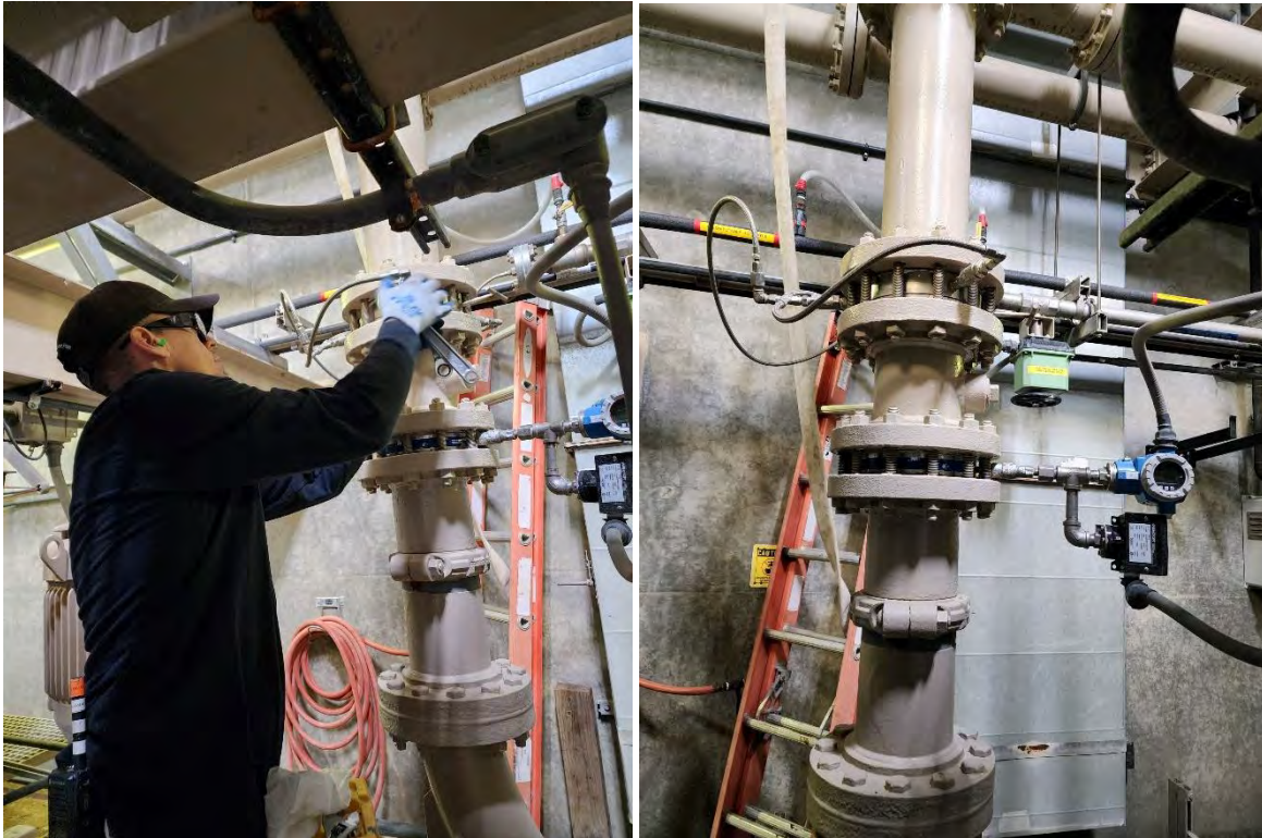
Staff removing injection check valves for cleaning (left); and injection check valves after cleaning (right) at the Weymouth plant
