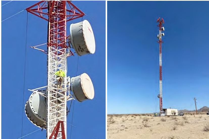
Staff repairing a microwave dish on a communications tower at a Desert facility
