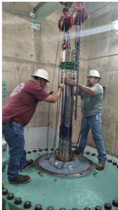
Staff test fitting the lift nut for a unit's discharge valve at Eagle Mountain pumping plant
