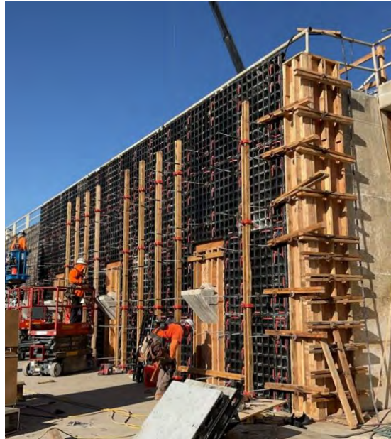
Weymouth Basins 5-8 and Filter Building No. 2 Rehabilitation —Fabrication of steel and formwork for Basin 8 drywall
