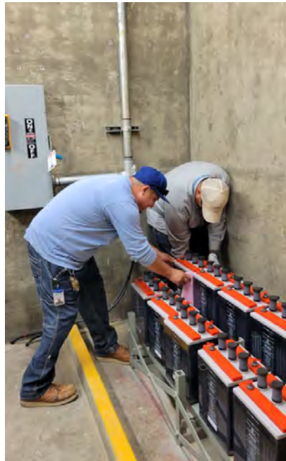
Staff setting batteries in place before making final connections at (Corona/Temescal HEP)
