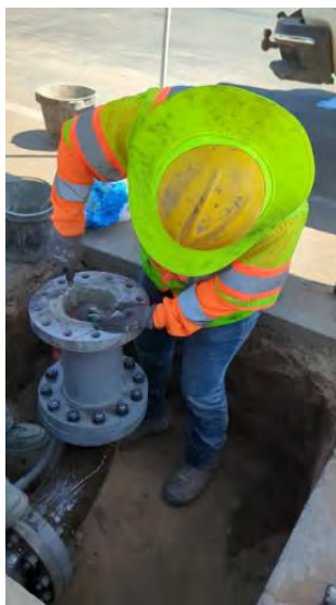
Orange County Feeder Lining Repairs — Installation of piping for new air release valve
