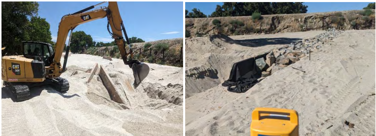
Staff excavating K-rail and steel plates (left) and new measures (right) in the San Jacinto River Crossing
