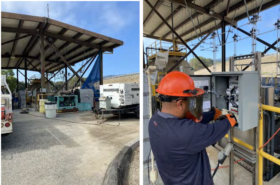
Test equipment set up for functional test (left); and staff taking readings (right) of critical equipment at Palos Verdes Reservoir
