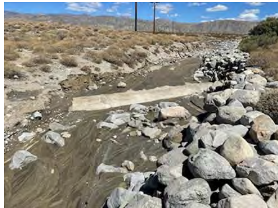
CRA conduit exposed along the CRA
