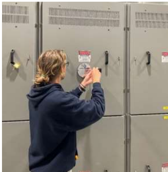
Staff installing infrared scanning windows onto high-voltage equipment at the Skinner plant
