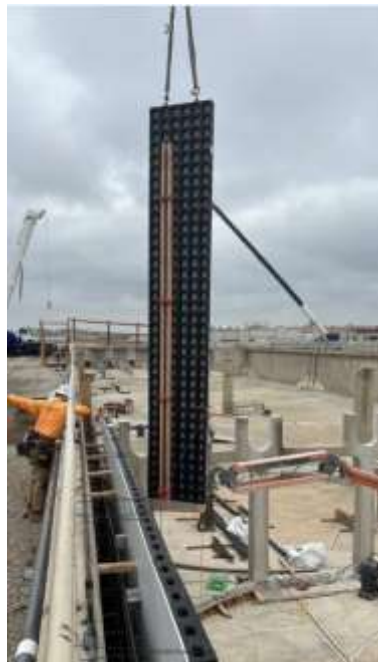
Weymouth Basins 5–8 and Filter Building No. 2 Rehabilitation Installation of Concrete Placement Panels
