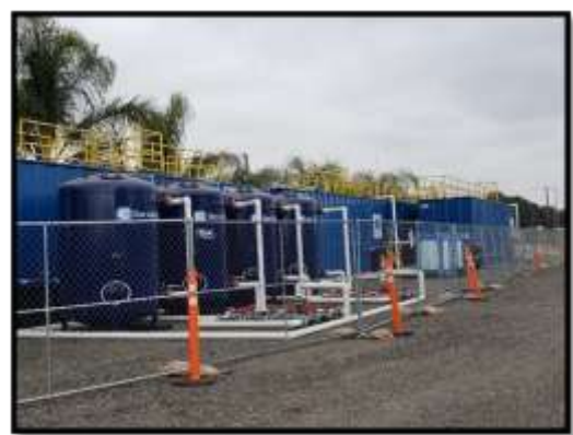
Granular activated carbon (GAC) treatment plant to filter groundwater for Perris Valley Pipeline Project
