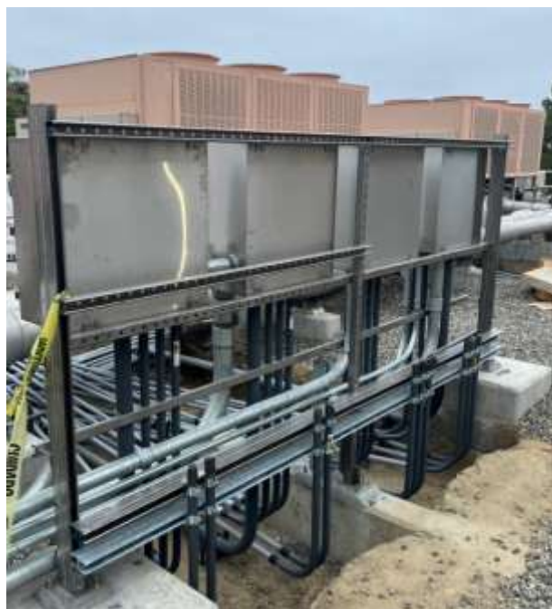
Figure 10C-88 Pump Station Chillers Replacement Electrical Conduit Installation
