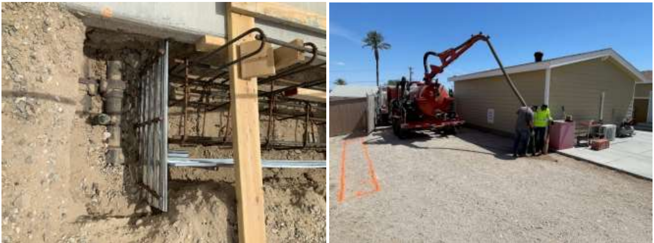
Footing formed to protect utility (left) and staff potholing buried utilities (right) at a Desert housing unit
