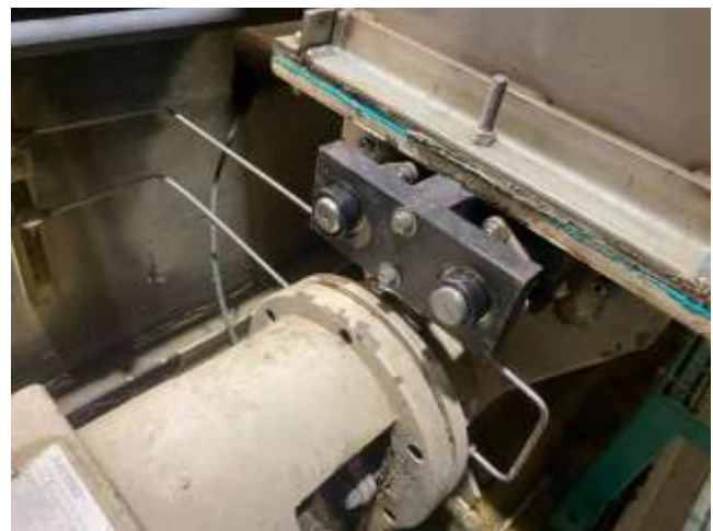
New bridge breakers (left) and bearings (right) on the sludge pump at the Diemer plant
