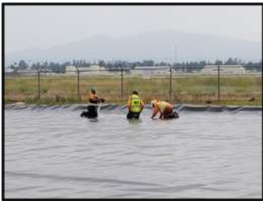
Construction contractor placing a liner for soil storage for Perris Valley Pipeline Project
