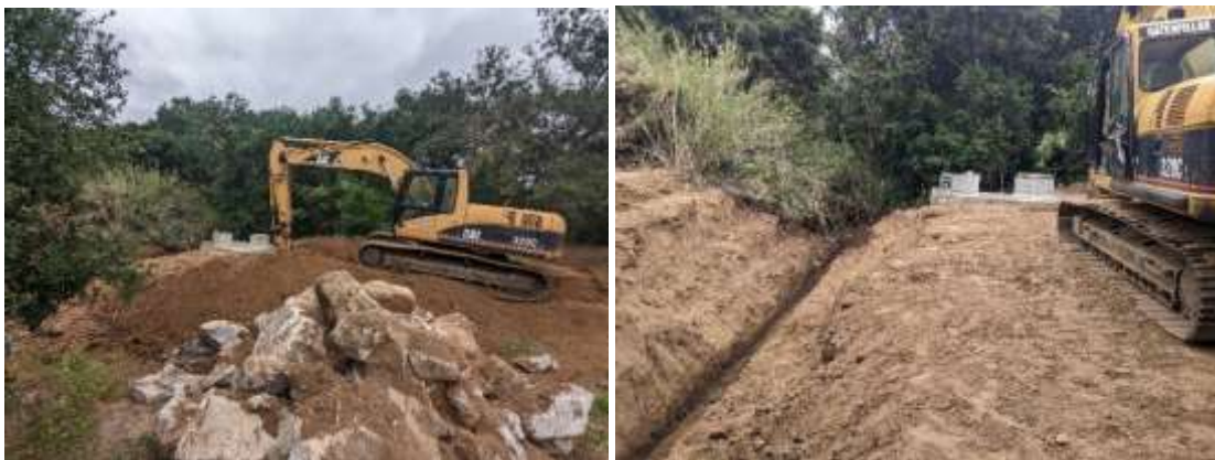
Staff using an excavator to complete the trench for the culvert along San Diego Pipelines 4 and 5
