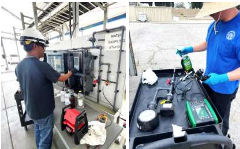
Staff troubleshooting instrument alarms (left) and calibrating pressures switches (right) at the Pure Water Southern California demonstration plant
