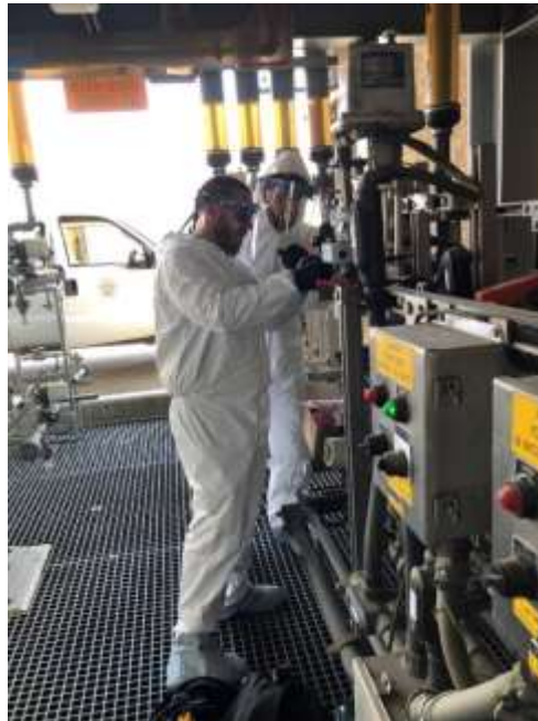
Staff installing a magnetic flow meter for measuring sodium hypochlorite at the Skinner plant
