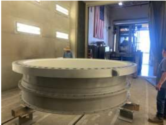
Coated upstream thimble (left) and downstream thimble (right) for the Upper Feeder repairs
