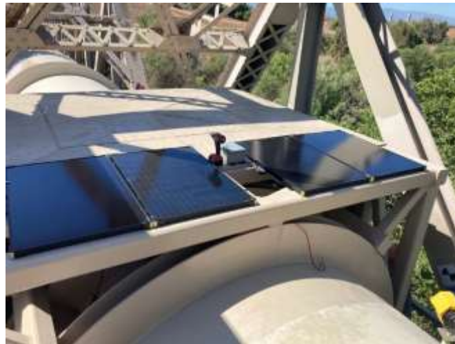
Solar panels for providing power to equipment monitoring sensors on the Upper Feeder's Santa Ana River bridge crossing
