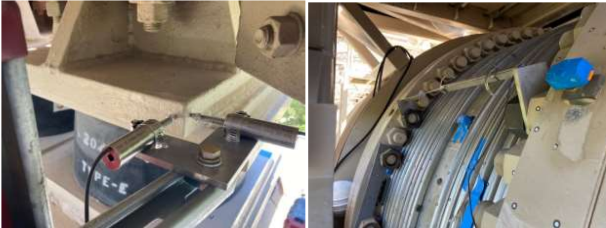
Equipment monitoring sensor installed at the Upper Feeder's Santa Ana River bridge crossing
