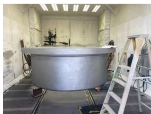
Blasting of the upstream thimble (left) and completed blasting of the downstream thimble (right) for the Upper Feeder repairs
