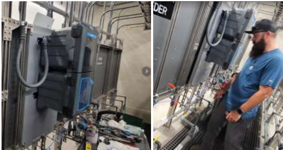
Staff installing sample line tie-ins to ammonia analyzers at the Weymouth plant
