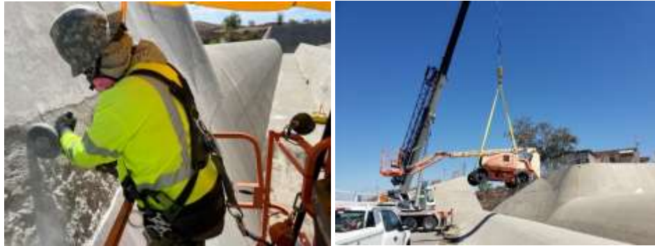
Staff removing loose and unstable material (left) and hoisting a man lift into the spillway channel (right) at Lake Skinner
