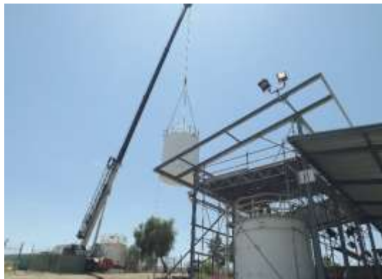
Staff using a crane to place the new sodium hypochlorite tank at Lake Mathews
