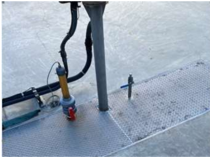
Ozone contactor afterbay gate hatch with a welded sample port at the Diemer plant
