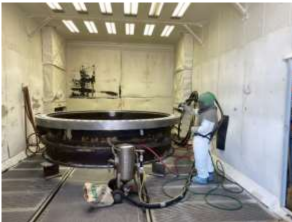
Blasting of the upstream thimble (left) and completed blasting of the downstream thimble (right) for the Upper Feeder repairs
