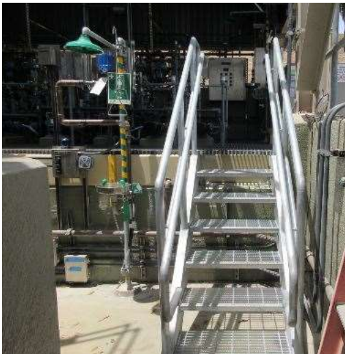
Garvey Reservoir Hypochlorite Feed System Replacement —New stairs for access to the containment area.
