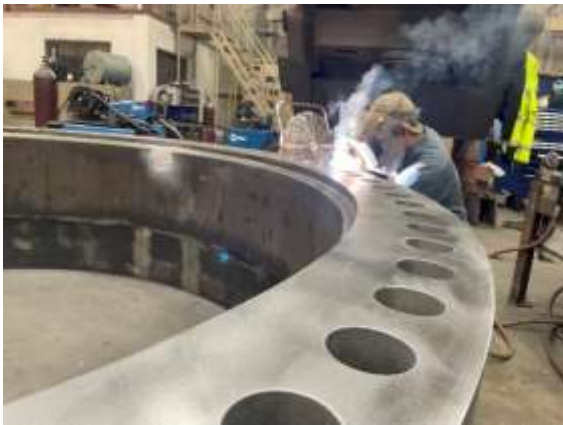
Staff welding flanges to upstream thimble (left) and downstream thimble (right) for the Upper Feeder repairs
