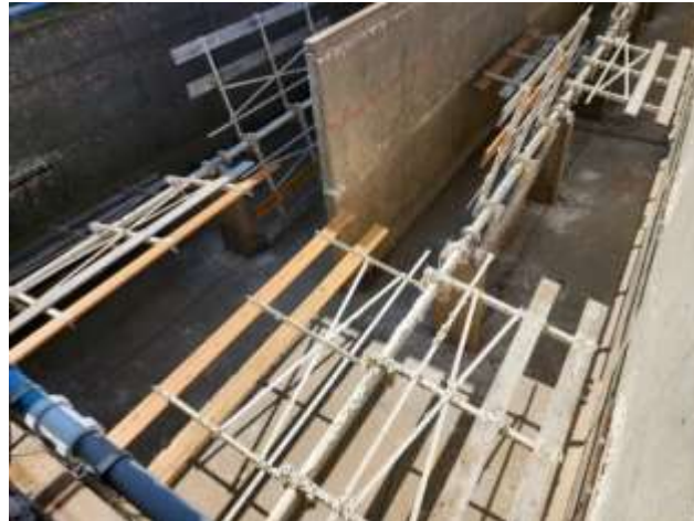
New sedimentation basin flocculator paddle boards at the Weymouth plant
