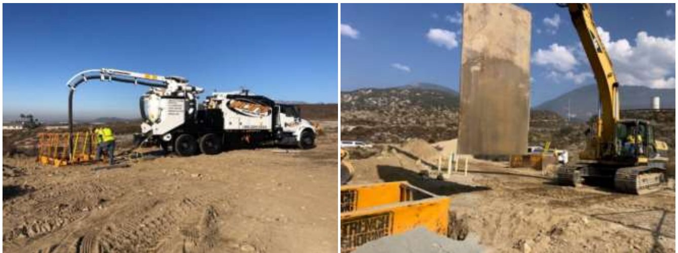
Potholing operations (left) and staff installing steel end plates (right) at DWR's Devil Canyon Facility
