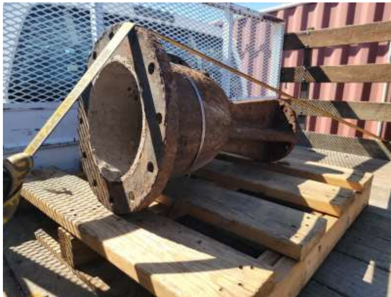
Before (left) and after (right) blasting and coating of circulating water pump components for Eagle Mountain pumping plant
