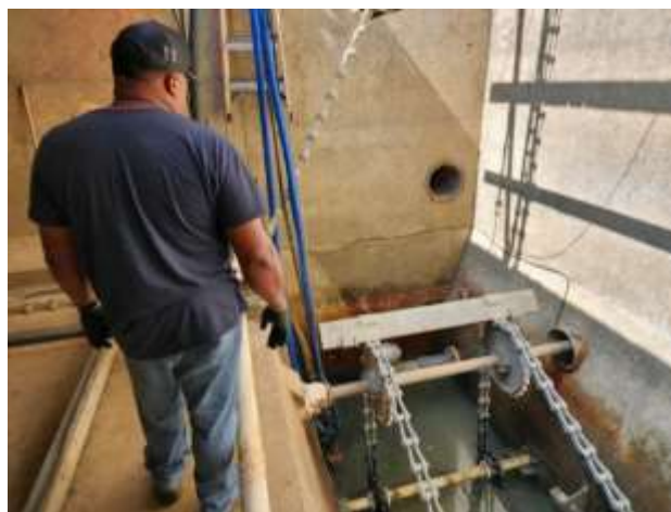
Staff dewatering a sedimentation basin at the Weymouth plant
