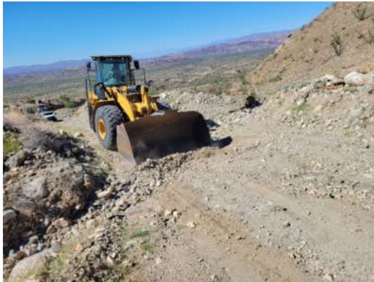
Staff repairing storm damage at the Chuckwalla communication site
