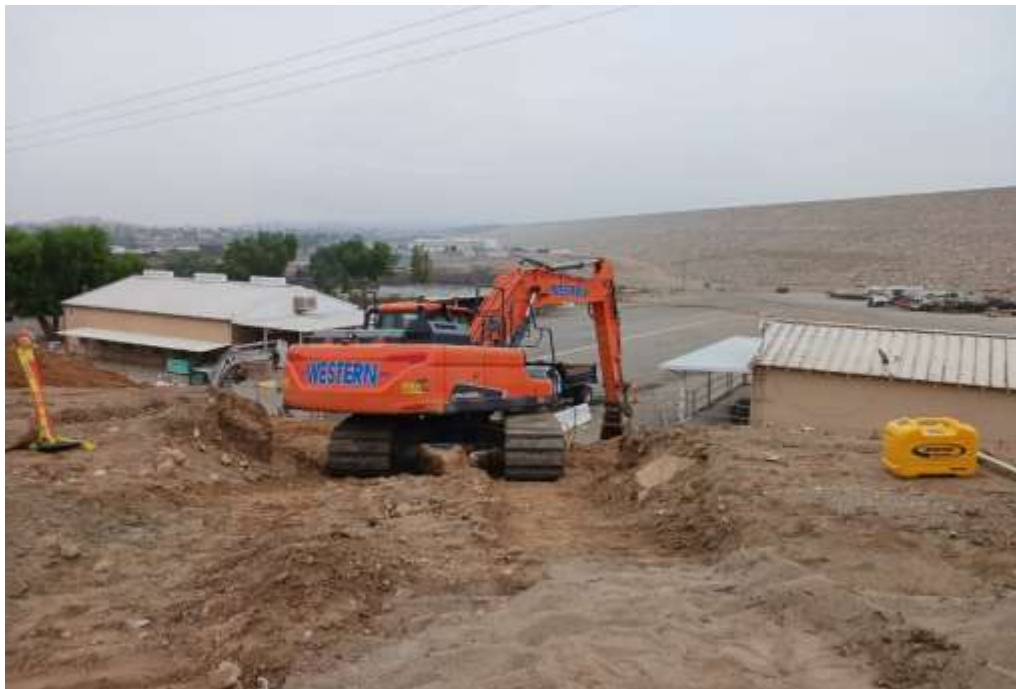
Lake Mathews Wastewater Replacement —Excavating sewer Line around the Lake Mathews Conference Room building
