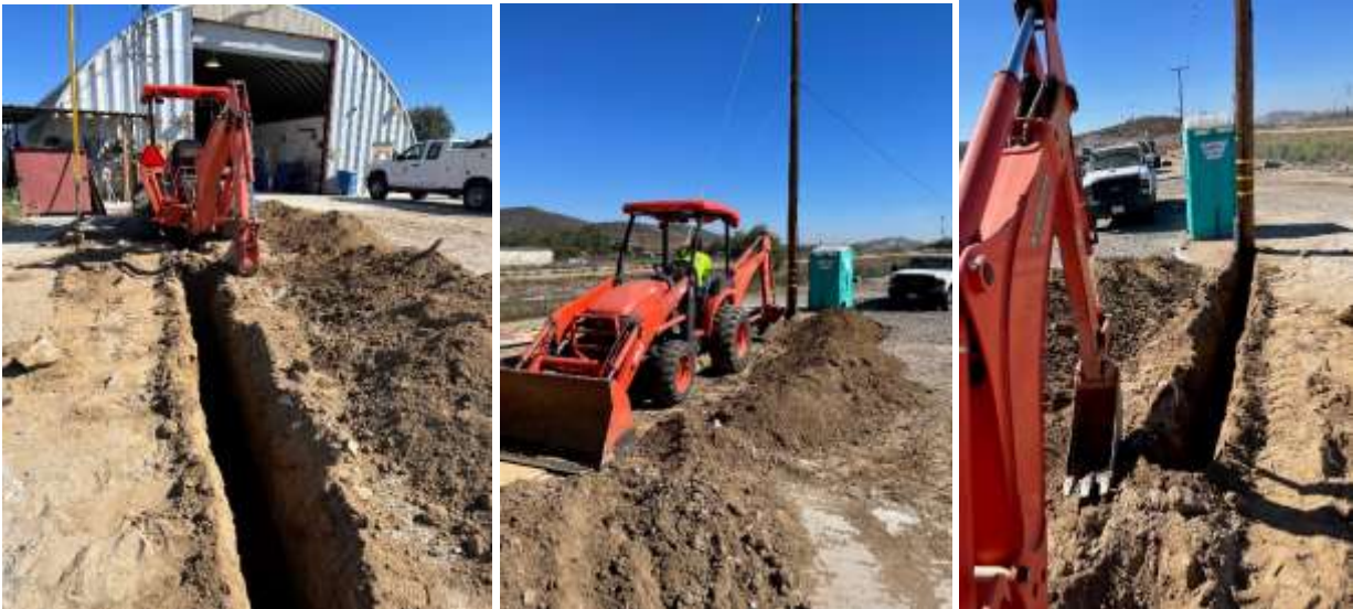
Staff trenching dirt to relocate an incoming overhead power line to an underground route at the DVL fleet shop
