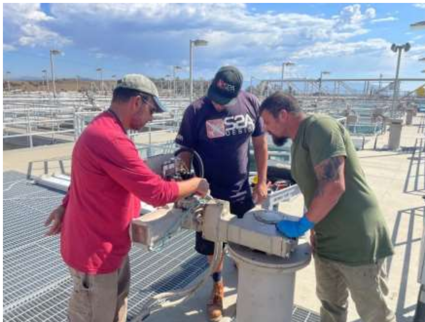
Staff installing the repaired filter drain gearbox at the Skinner plant
