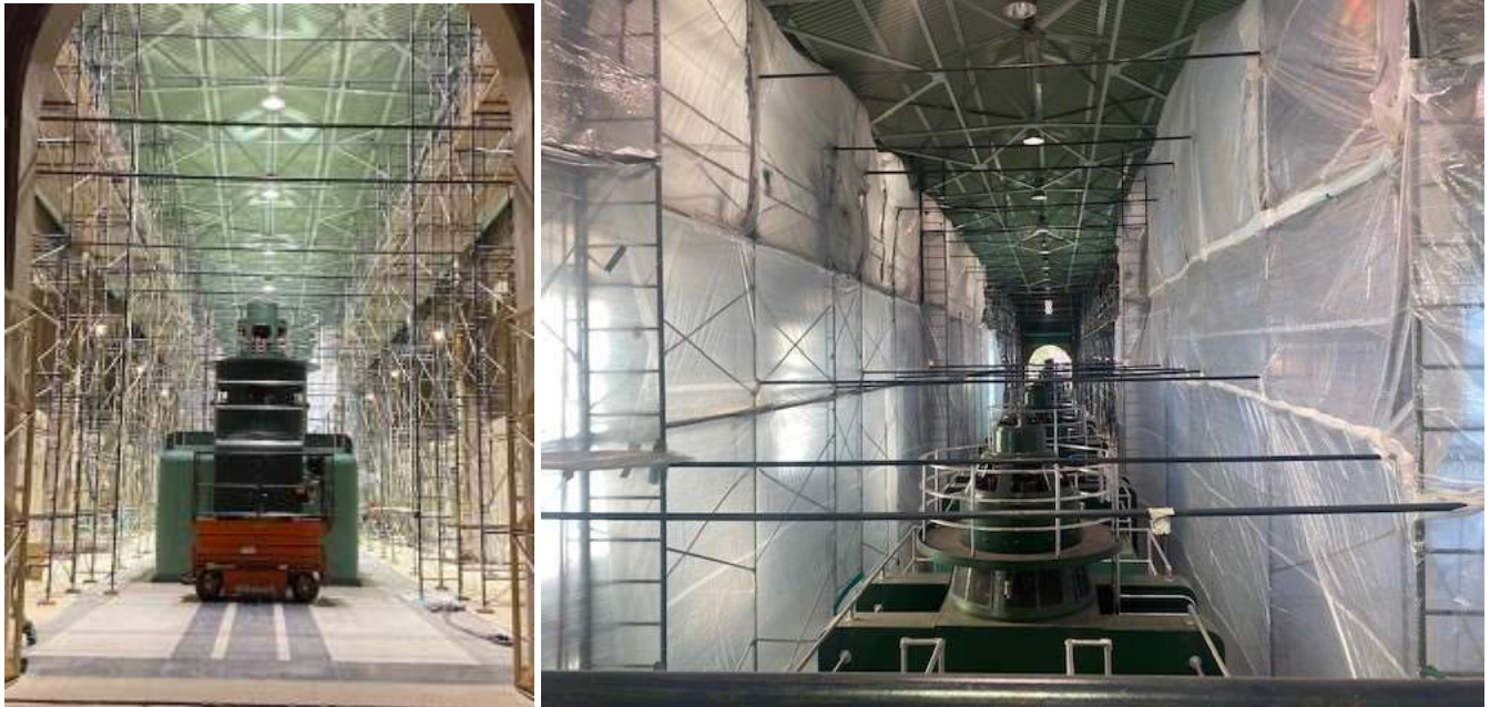
Overhead crane replacement at Gene pumping plant
