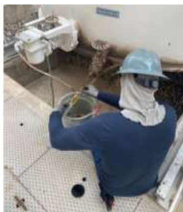
Staff taking an oil sample from a transformer at Gene pumping plant
