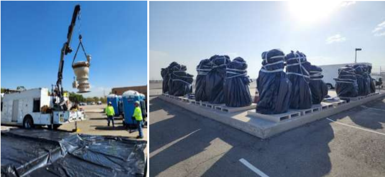
Off-loading (left) and palletizing valves (right) to be stored during phase 3 of the Etiwanda Pipeline relining
