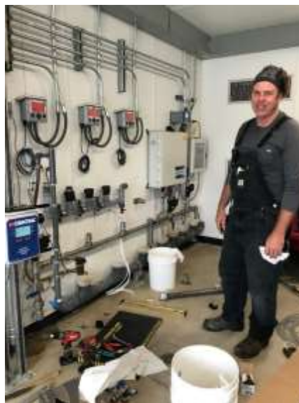
Kenneth Lorenzo (Jensen O&M Tech IV) installing the modified analyzer probe manifold at the Jensen plant
