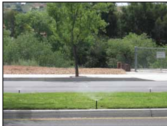
(Pictured left) Discharged wastewater from industrial cooling towers is tested on California Friendly plants for irrigation. (Pictured right) Sprinklers with pressure reducers minimize runoff on greenbelt medians.
